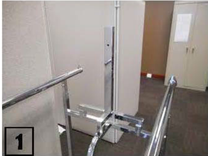
Saddle "Upright Bracket" over the existing H-Rack
