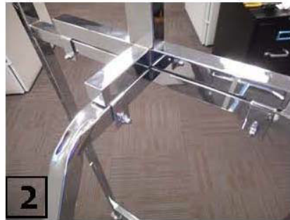
Once The "Upright Bracket" is in place it will need to be secured with a nut and bolt (included).
