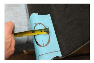
42. After cutting out your marked oval in the carpet and foam backing, make a straight cut from the outside edge of the oval to the outside edge of the carpet piece. This allows for installation.
