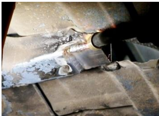
Figure 43 – Weld Back of Connector
