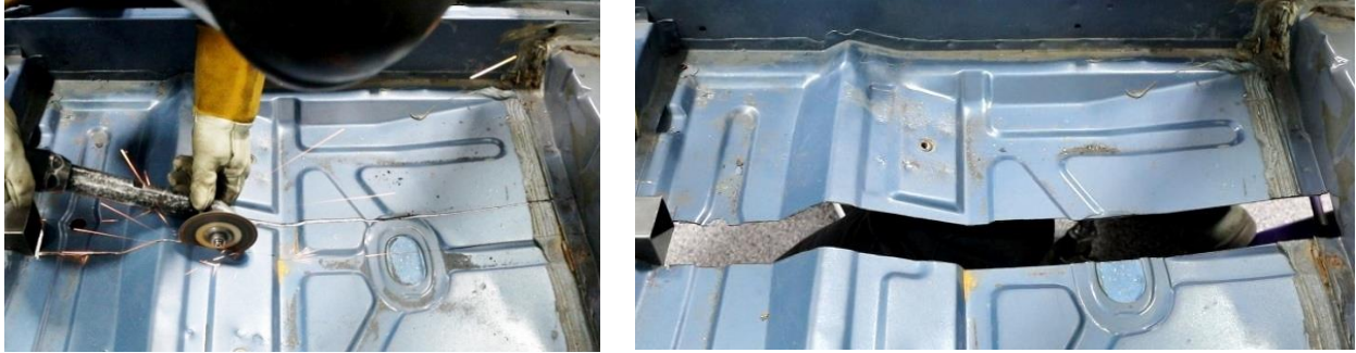
Figure 25 - Cut Floor Pan
