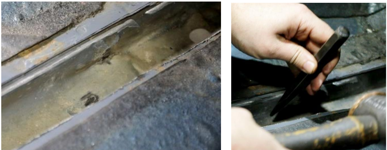
Figure 21 – Grind Away Burrs
