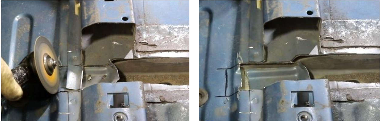
Figure 19 – Remove Floor under Seat Riser
