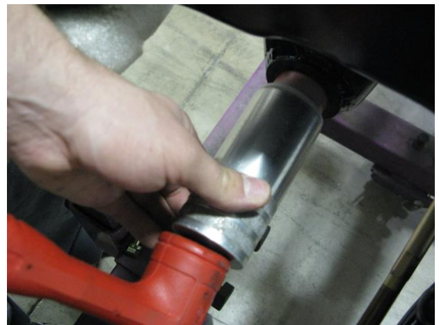
Figure 6 - Fully Installing the Bushings
