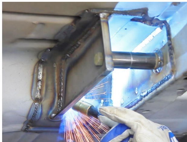
Figure 10 - Weld Inboard Plate
