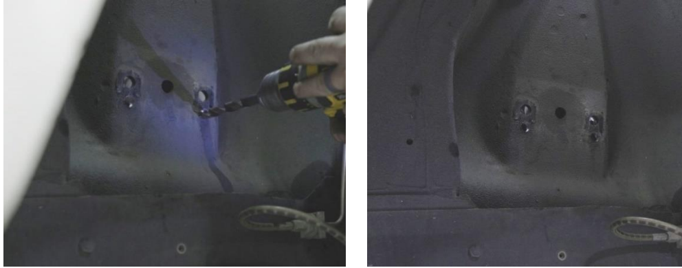
Figure 5 - Drill Mounting Holes
