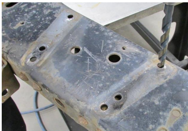
Figure 18 - Drill Out Frame Holes
