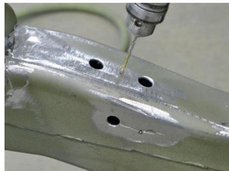
Figure 47 – Drill & Chamfer Nut Plate Locators
