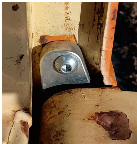
Install top fastener
