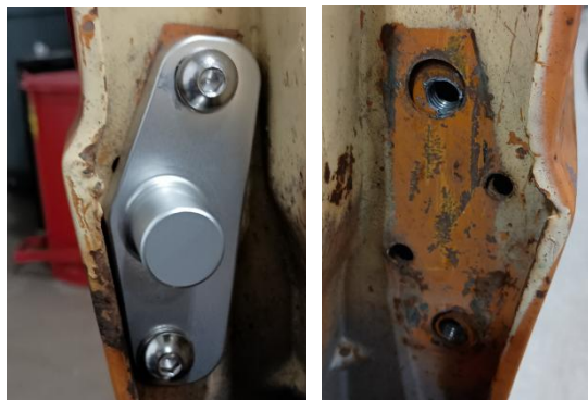
Install Trunnion Base, prepare for tailgate installation
