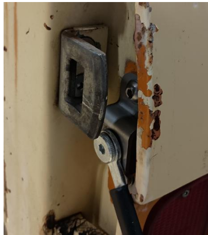
Install Latch Bracket
