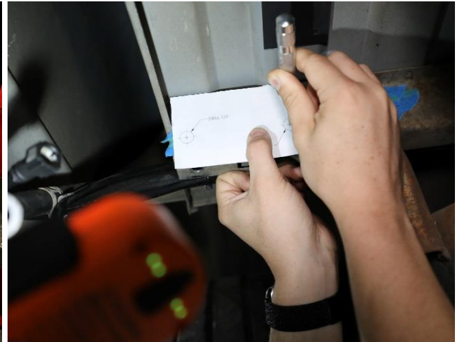
Figure 2 - Mark Holes Using Drill Template
