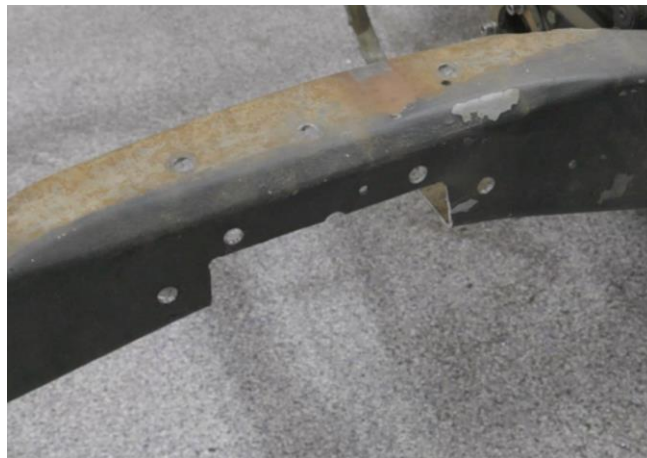
Figure 15 - Drill Holes for Frame Notch
