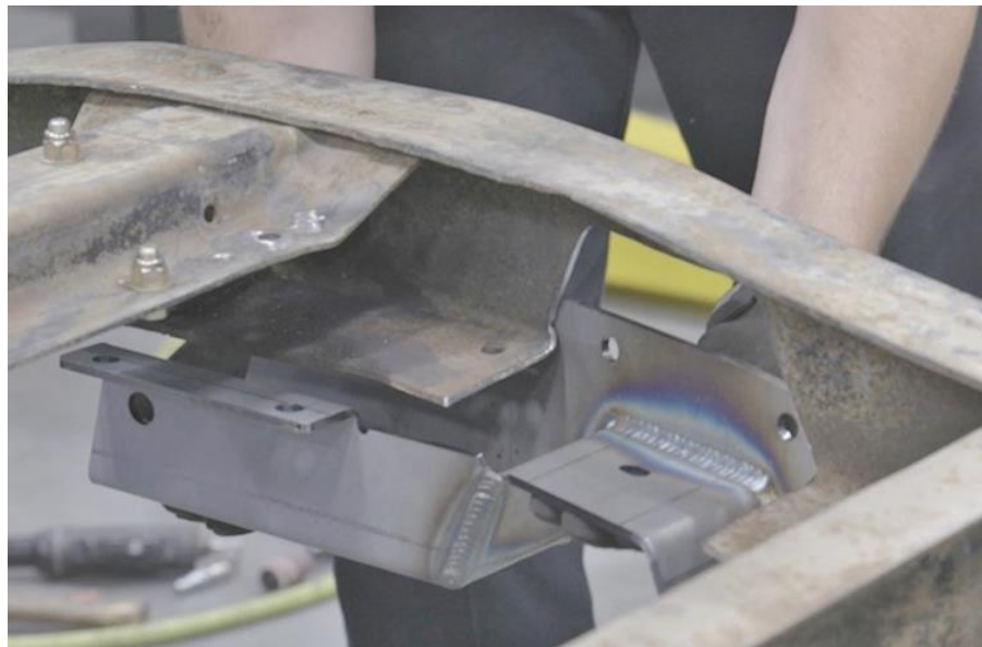
Figure 15 - Test Fit Frame Notch Assembly
