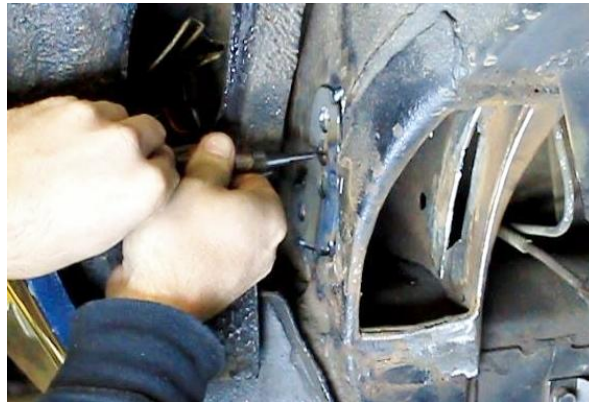
Figure 13 - Center Punch Trailing Link Holes
