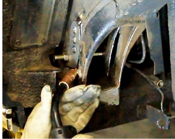
Figure 12 - Tack Weld Doubler Plate
