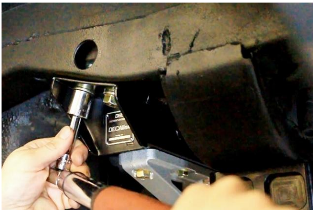
Figure 85 - Torque 1/2"-13 Hardware
