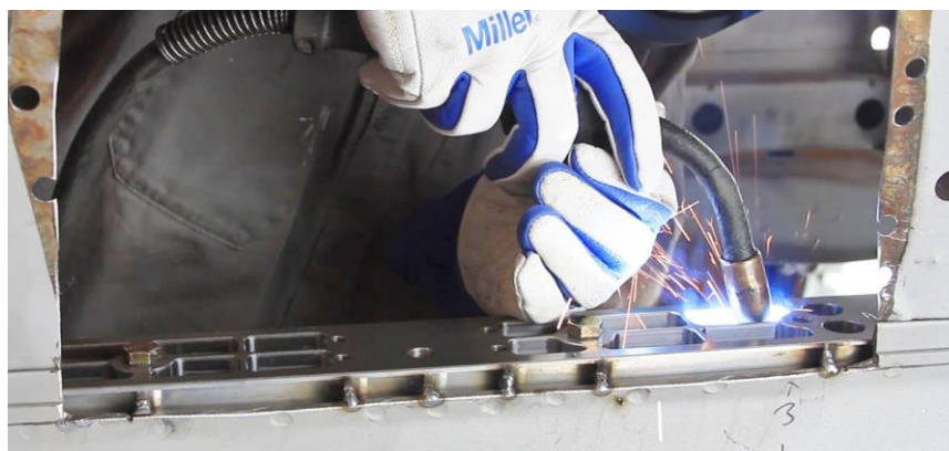
Figure 17 - Finish Weld Adapter Plates & Floating Stanchions
