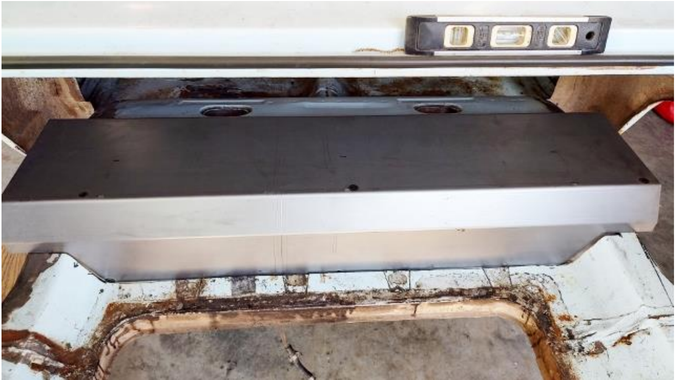
Figure 5 - Test Fit Crossmember
