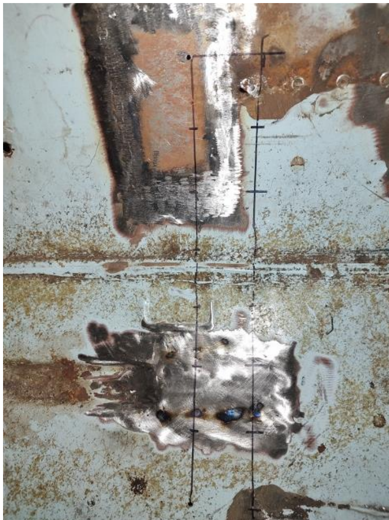
Figure 14 - Mark Plug Weld Locations
