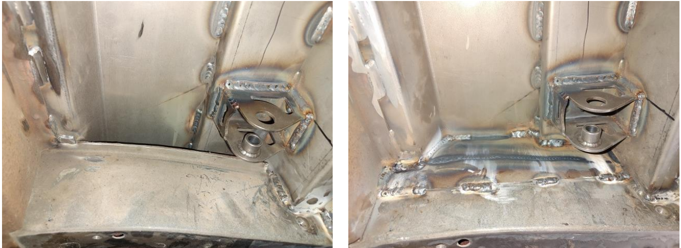
Figure 9 - Weld Closeout Plates
