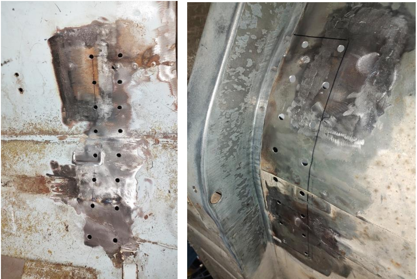
Figure 15 – Drill Plug Weld Holes
