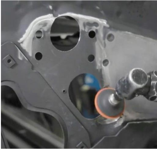
Figure 5 - Prep Firewall for Welding
