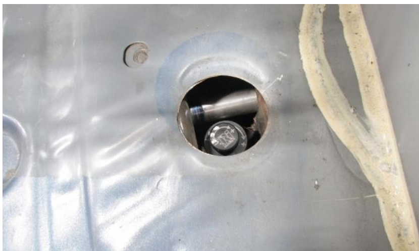
Figure 43 - Trunk Floor Access Hole
