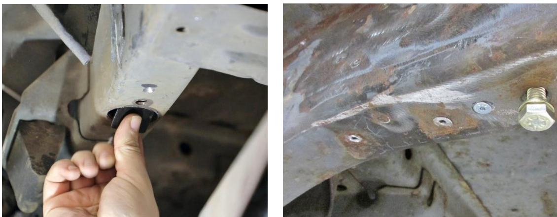
Figure 30 - Install Weld Nut Doubler Plates
