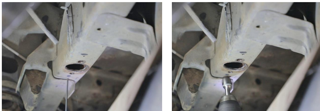
Figure 29 – Drill & Chamfer Nut Plate Mounting Holes
