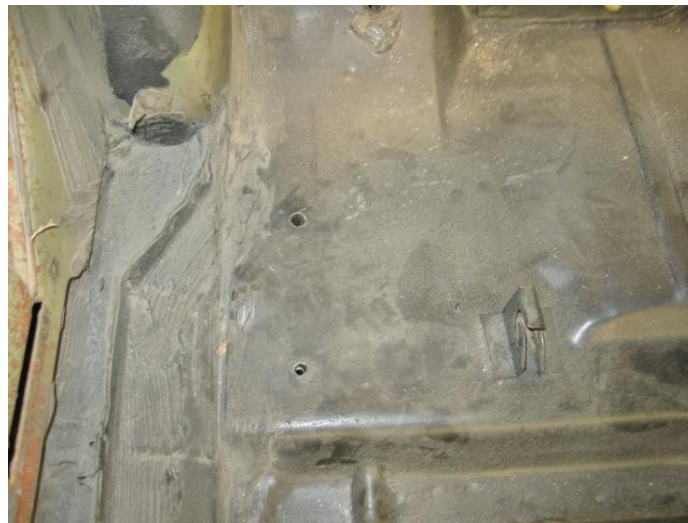
Figure 6 – Drill Location Holes
