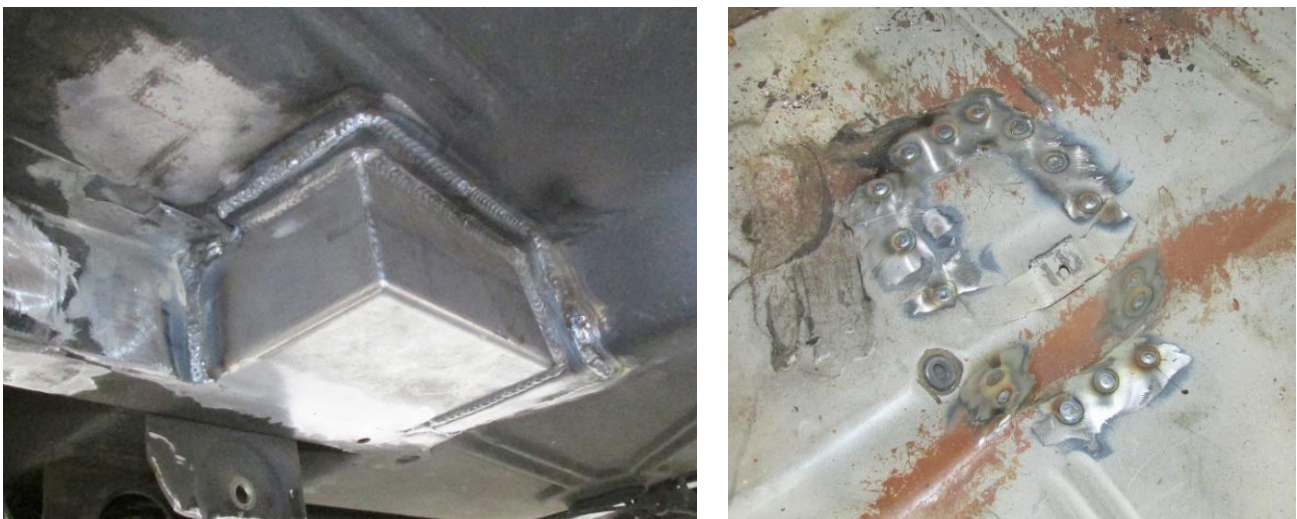
Figure 9 - Weld Torque Boxes
