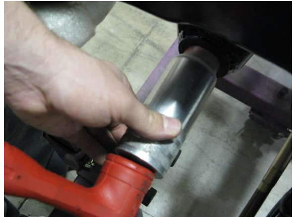
Figure 7 – Fully Installing the Bushings
