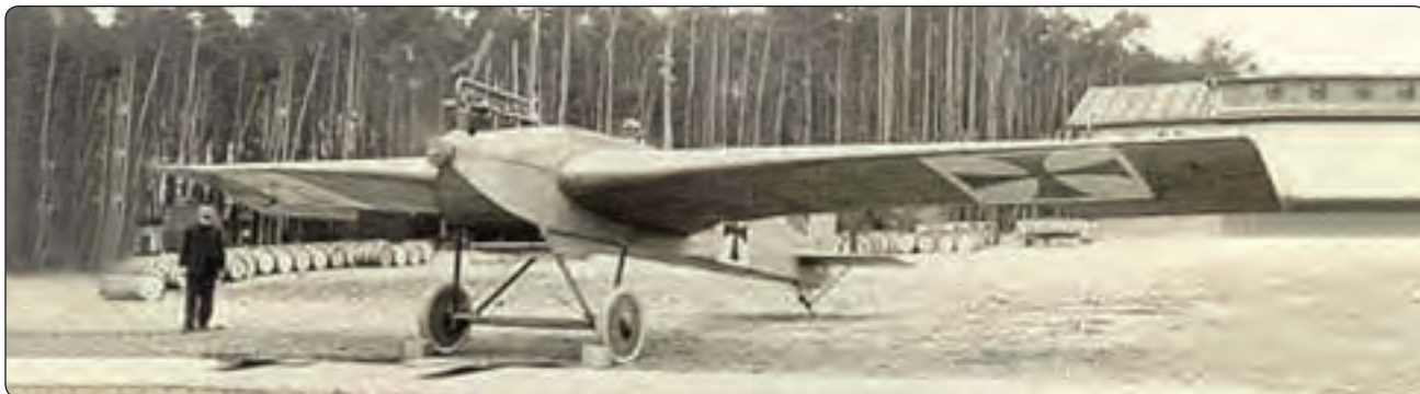
Figure 1-6. The Junker J-1 all metal construction in 1910.
