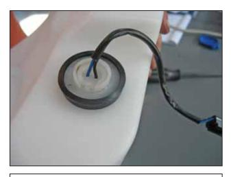
p. Apply a liquid soap solution to the level sensor and insert it into the grommet. Make sure that the level sensor is pressed all the way into the grommet. The lip of the sensor should sit inside the groove of the grommet.
