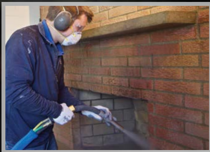
Wood and Brick Cleaning
