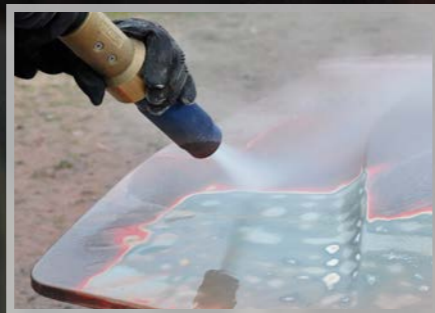
Coating and Paint Removal
