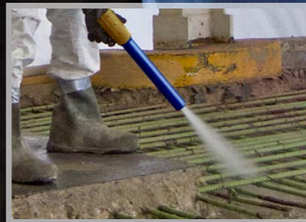
Concrete Repair and Restoration
