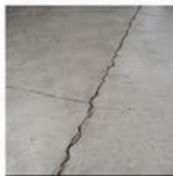
CONCRETE REPAIR PROJECTS
