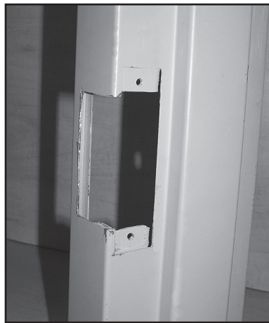
Frame Preparation: Should the frame not be cut out for the F1114, follow the directions located in Fig 3 on Page 2.
