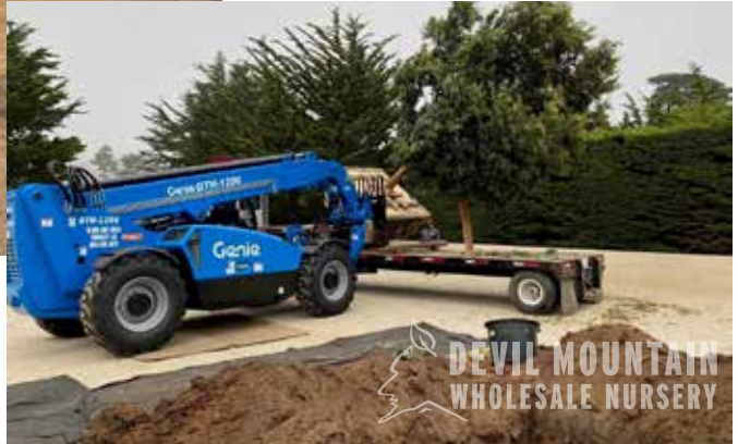
Offloading a 72" box with a telehandler
