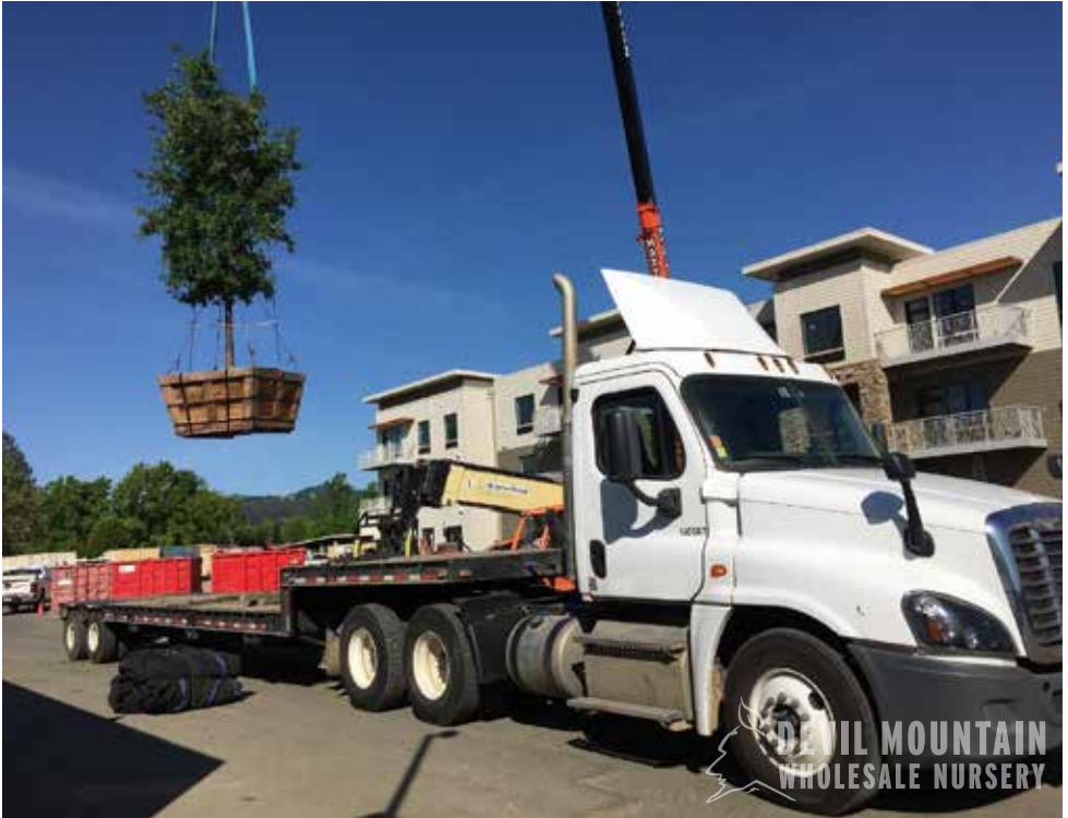
Crane offloading a 60" box tree
