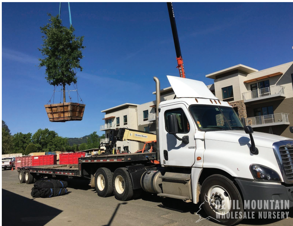
Crane offloading a 60" box tree
