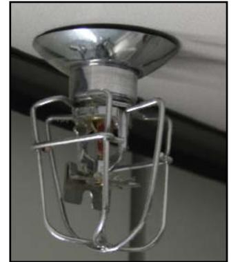
Designed to provide protection against low level impacts to the sprinkler head.
