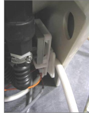
**Symptom: The toilet will not flush. Blockage at funnel on floor.**
