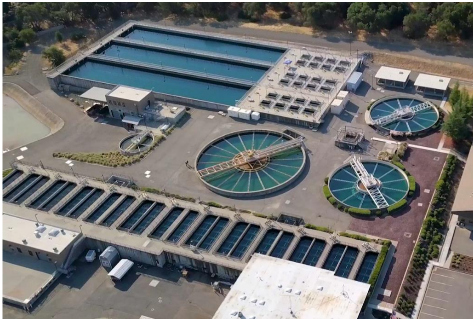
Figure 3: Aerial photo of a WTP. In the center are circular lime softener clarifiers. At the bottom is a row of sand filters. At the top are chlorine contact chambers.
