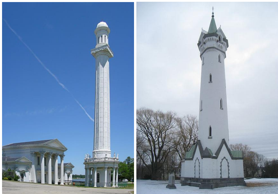
Figure 6: Examples of standpipe installations.
