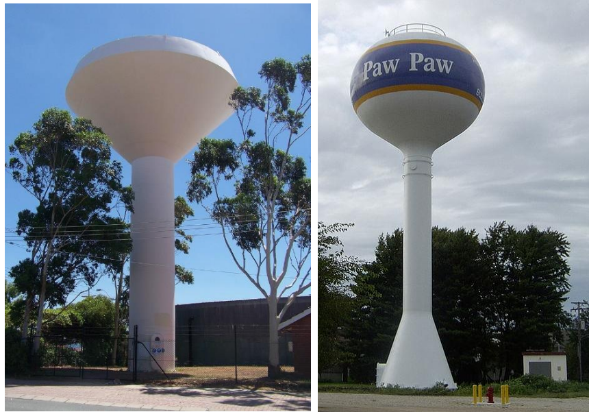
Figure 3: A conical bottom water tower (left) and spherical bottom water tower (right).
