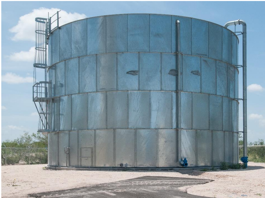
Figure 1: A stainless steel ground storage tank
