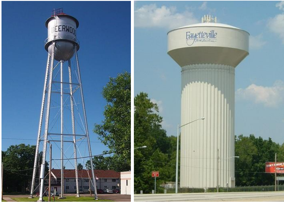
Figure 4: A multi-leg water tower (left) and a fluted column water tower (right).
