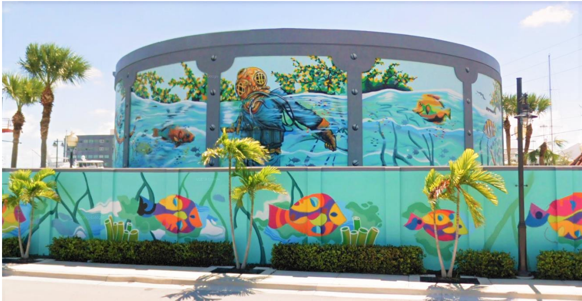
Figure 2: A concrete ground storage tank with pleasant architectural features.
