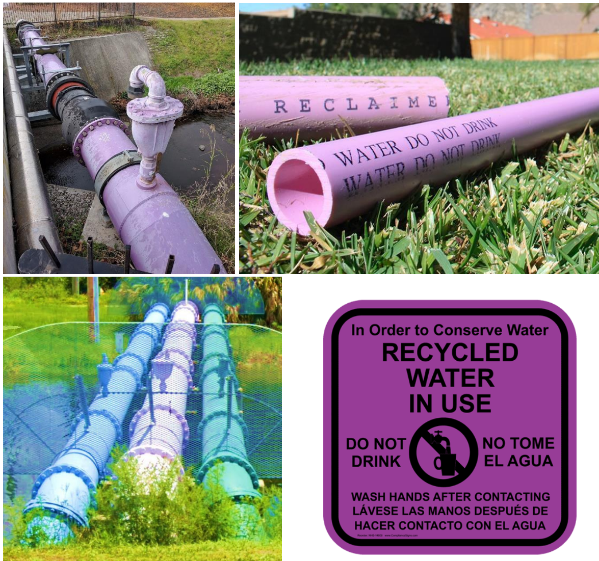
Figure 13: Upper left: A purple pipe in Mountain View, CA. Upper right: Reclaimed pipes with labels. Lower left: Portable main (blue), reclaim main (lavender), & force main (green).
