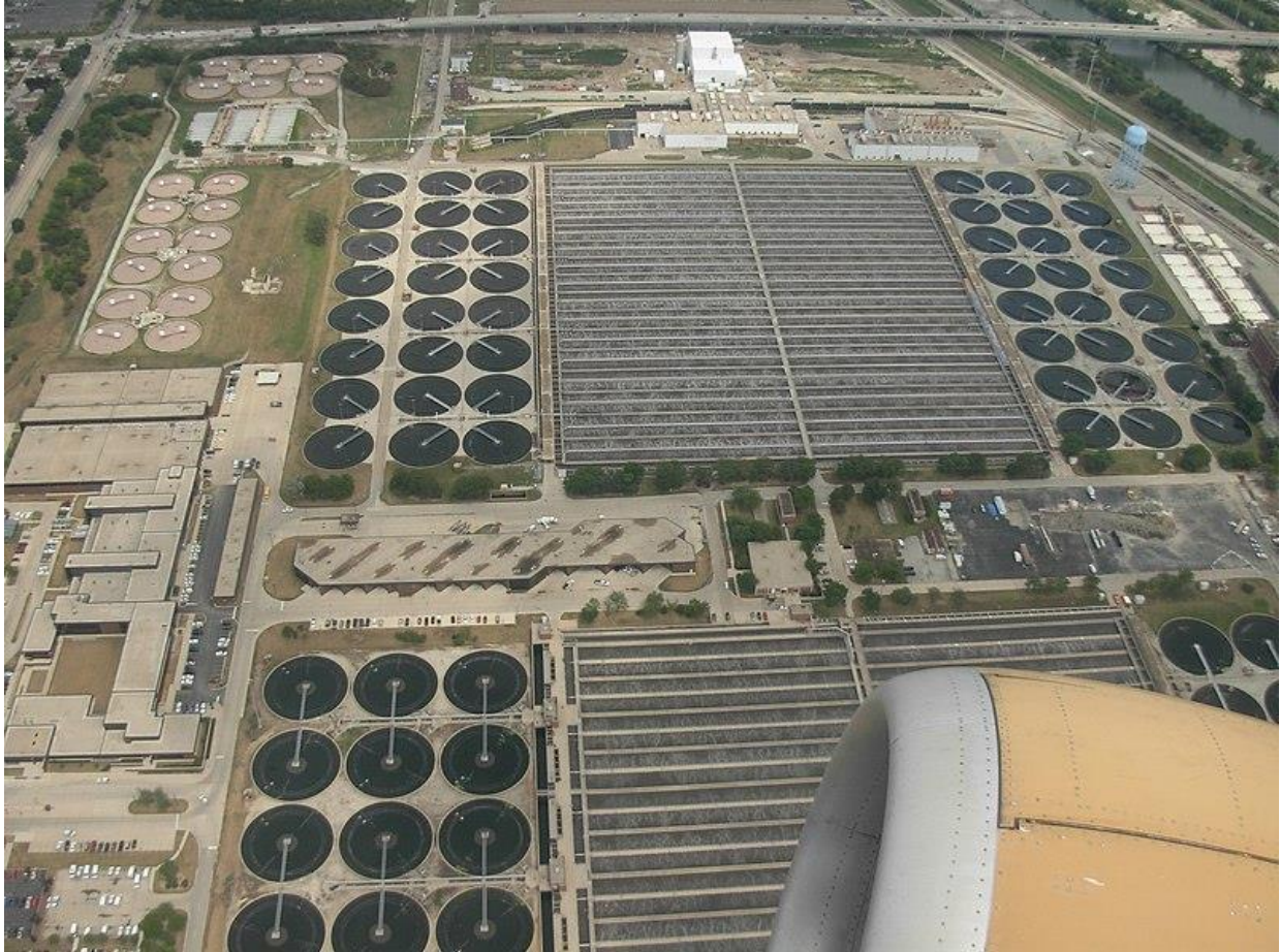
Figure 3: Stickney WRP in Chicago, considered the largest WWTP in the world. The wide rectangular tanks have aeration for biological treatment. The circular tanks are primary and secondary clarifiers.
