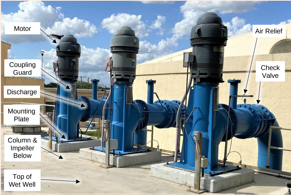
Figure 5: Three axial flow pumps mounted on top of a wet well for transferring water to a storage tank. An axial flow pump is similar to a mixed flow pump, as shown in Figure 4, except it has an axial flow impeller as shown in Table 1.
