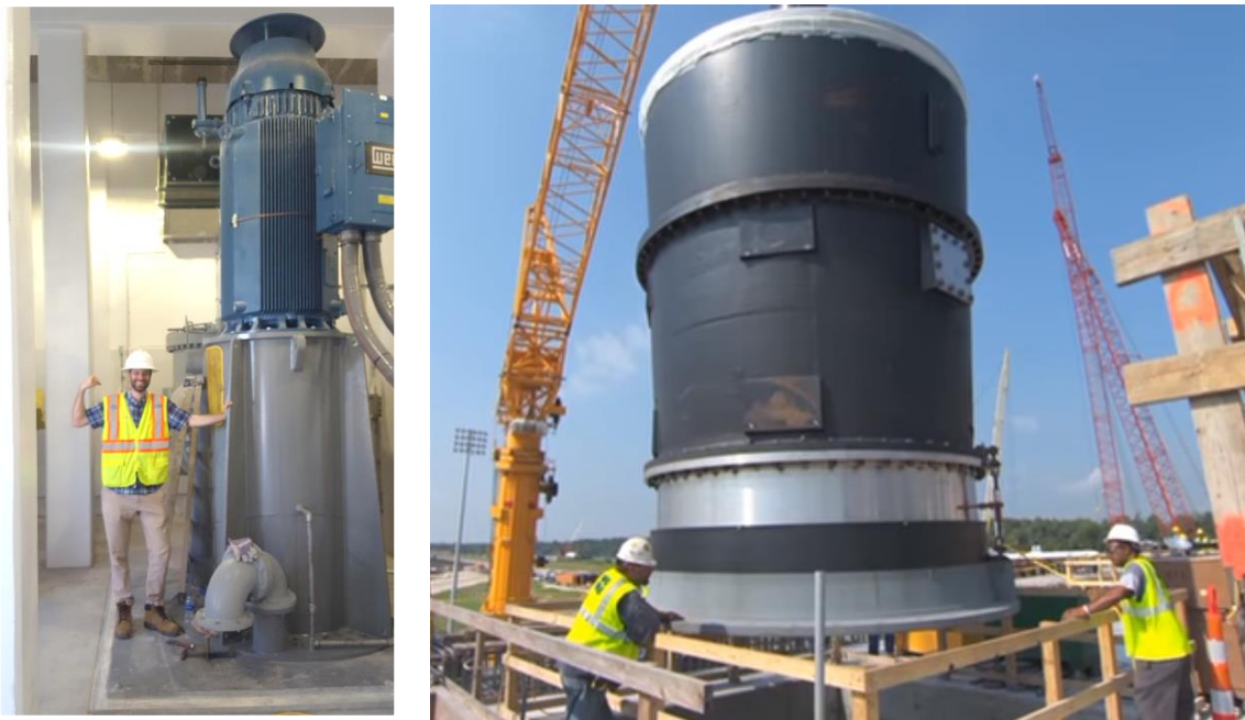
Figure 1a: Left: Author next to the top of a large vertical pump for moving canal water. Right: The lower section of an 11' dia. vertical pump for flood protection.
