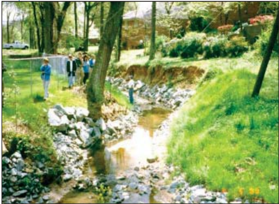
Figure 5.15 Channel armoring using riprap at the toe of the streambank
