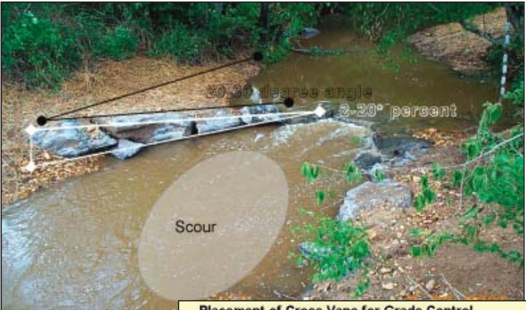
Figure 8.8 Cross vane showing placement and measurements * The lowest slope is most desirable, but in small streams a narrow channel may necessitate higher slopes (10 to 20 percent).
