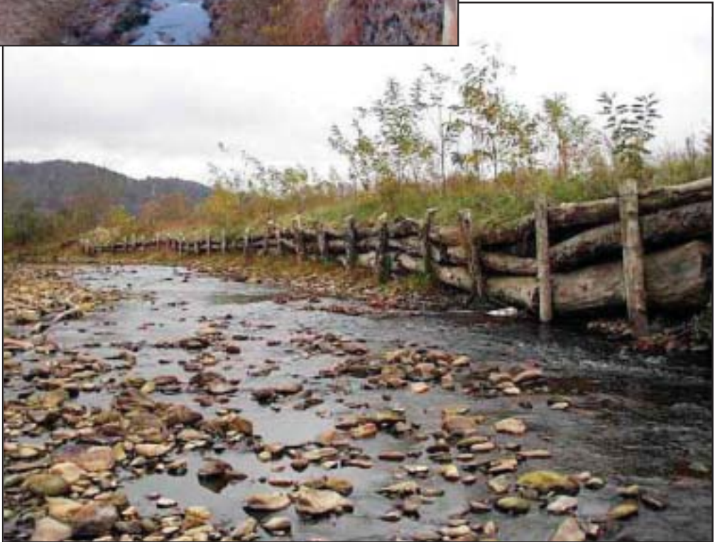
Figure 5.17 Armoring of streambank using log-crib wall
