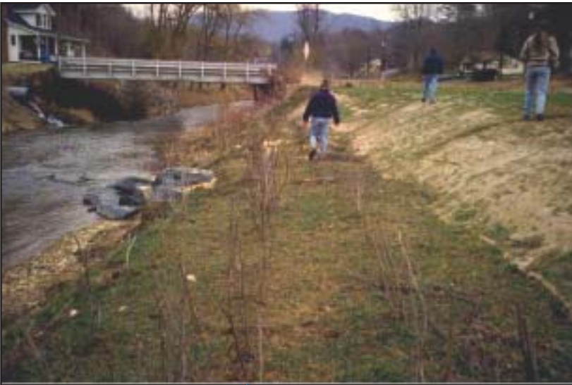
Figure 3.8 Bankfull bench on restoration site
