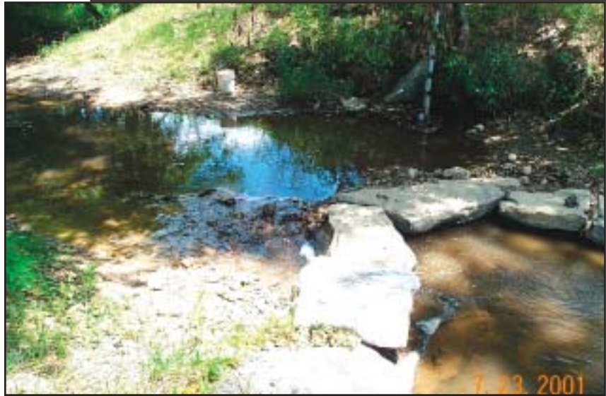
Figure 8.10 Hole formed on cross vane due to gap in structure
