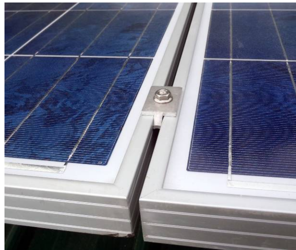
Close-up views of the installation of the solar panel, bolt, clamp, and nut
