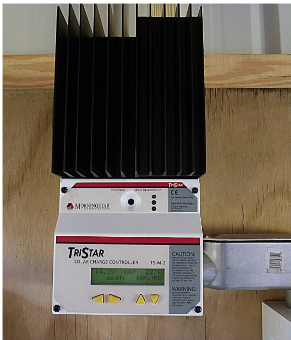
Behind the panel of the Morningstar TS-45 MPPT Charge Controller
