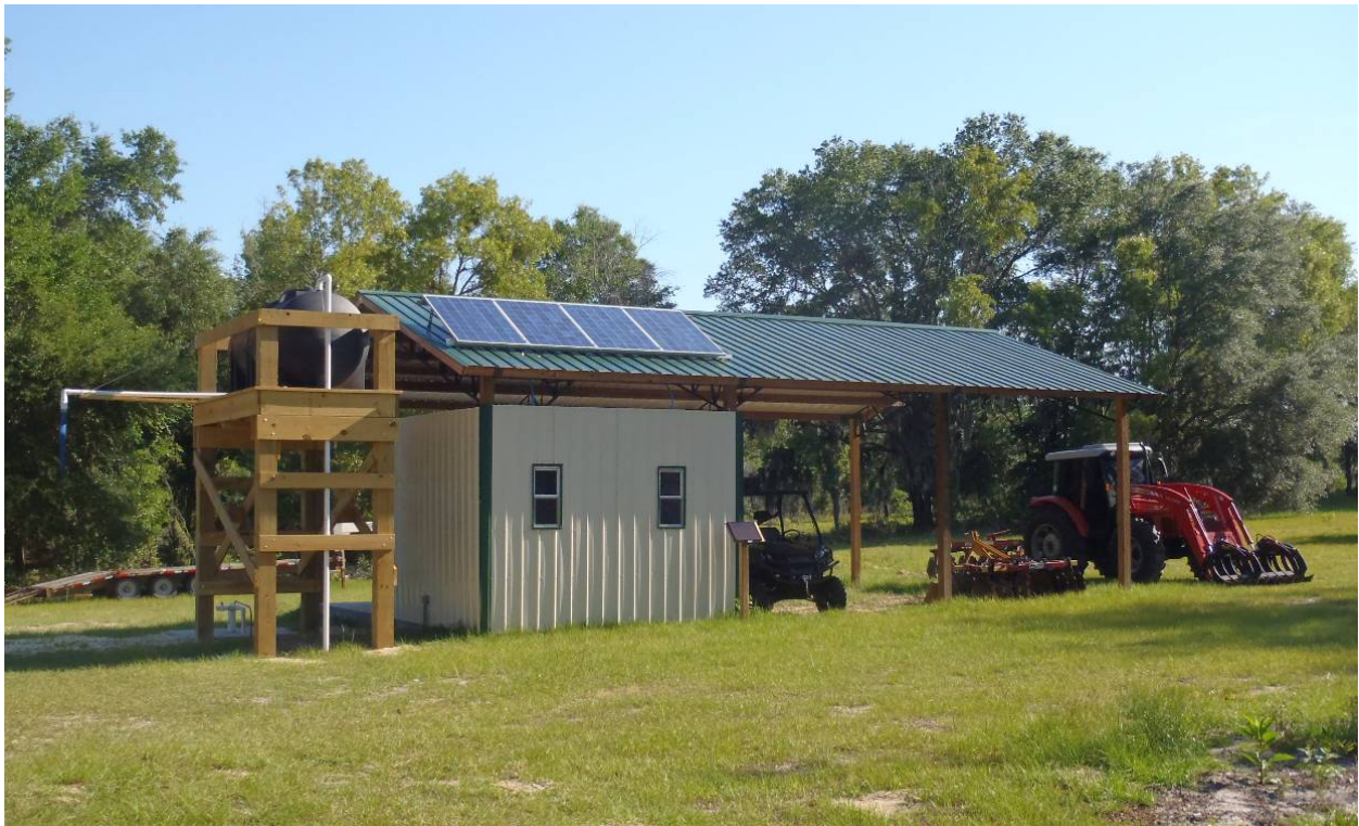
An off-grid solar powered shop and fire fighting water well
