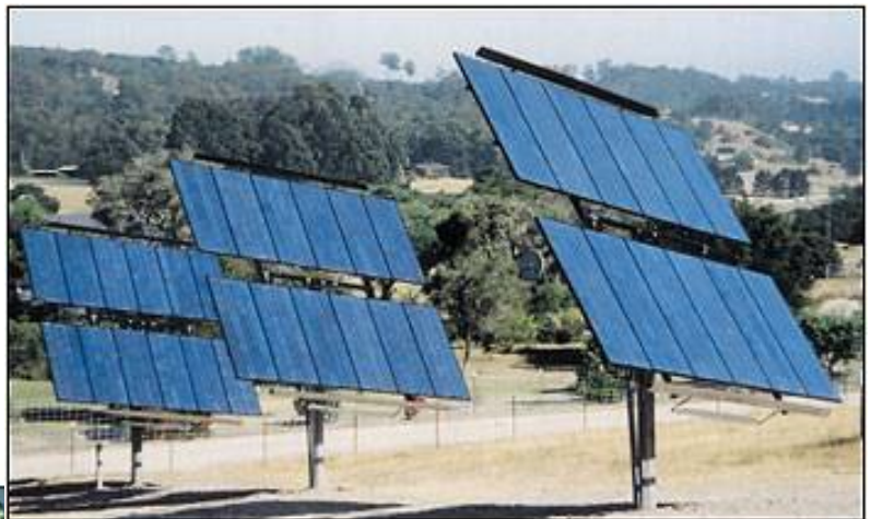
Zomeworks UTR-F 120 Track Rack™ by Renewable Energy Concepts
