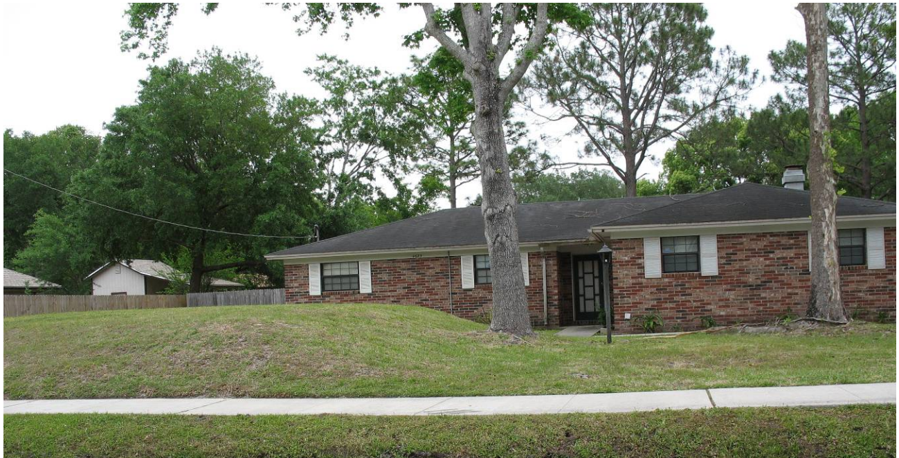
A residential mounded septic system
