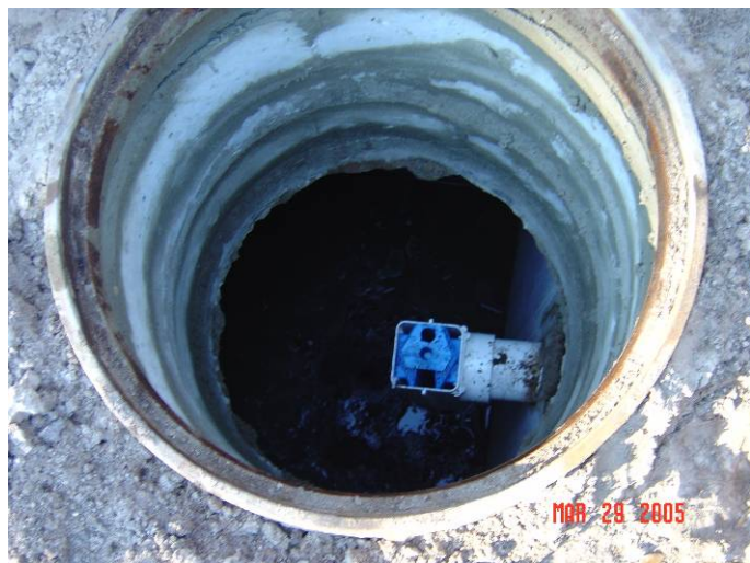
Filter access through manhole
