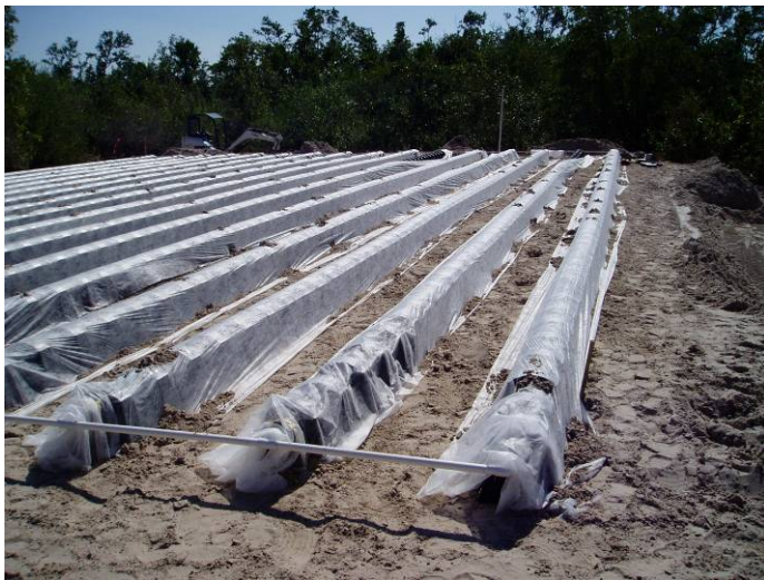
Septic drainfields using the septic chambers
