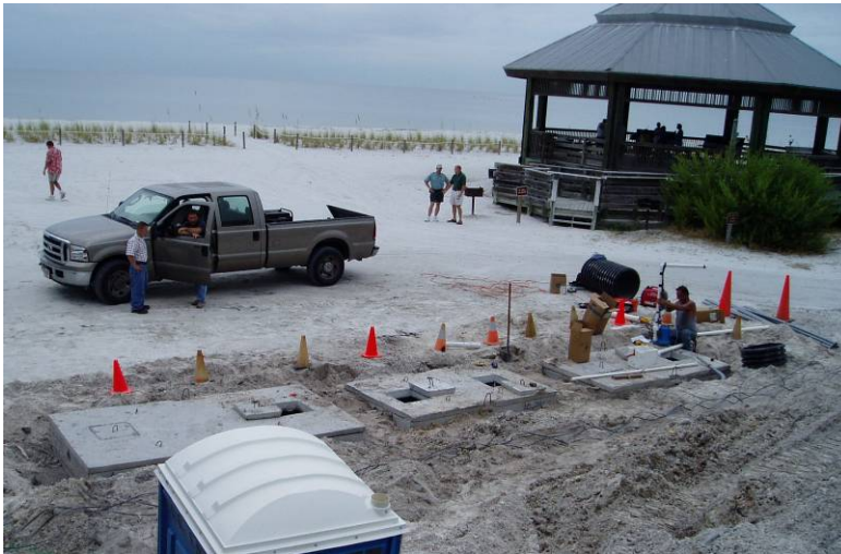
Septic Tank Installations
