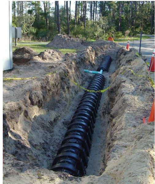
Septic drainfields using the septic chambers
