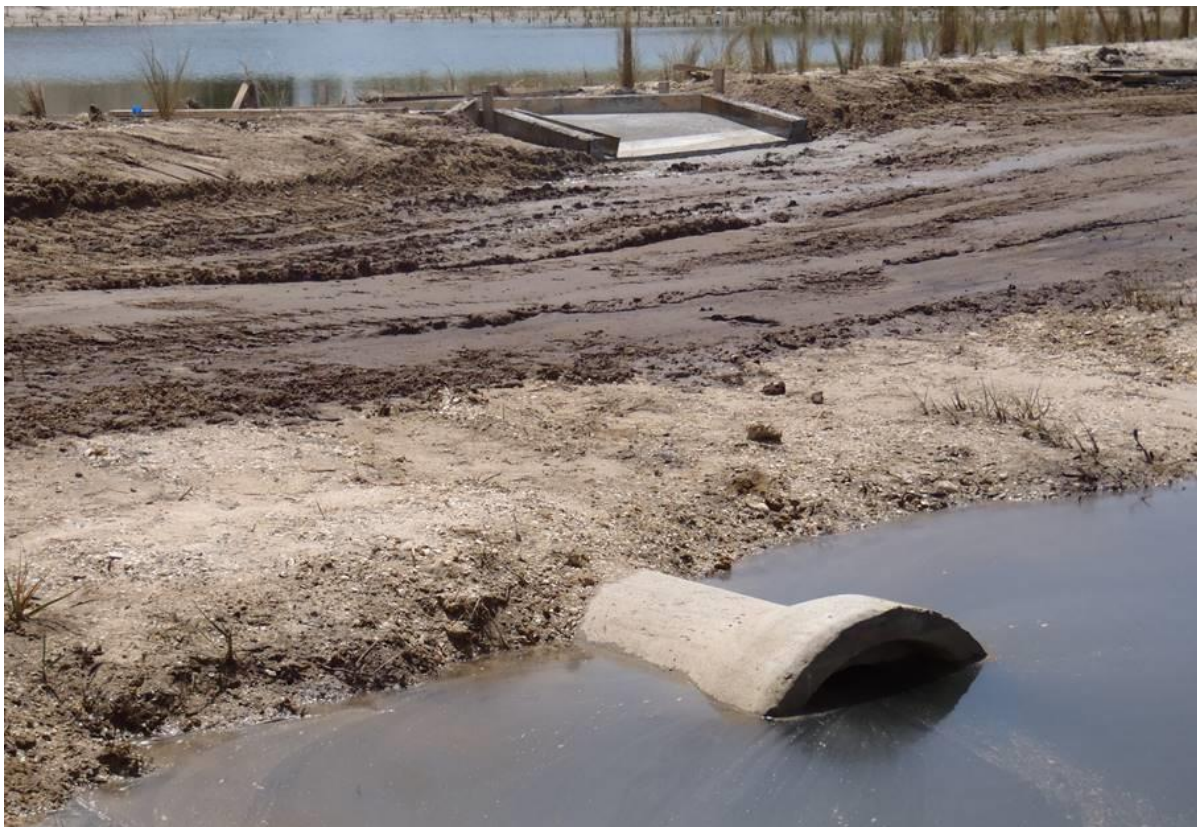
Figure 8 – Concrete culvert connection through berm to pond (the Spillway over the berm and into the Pond is in the background)
