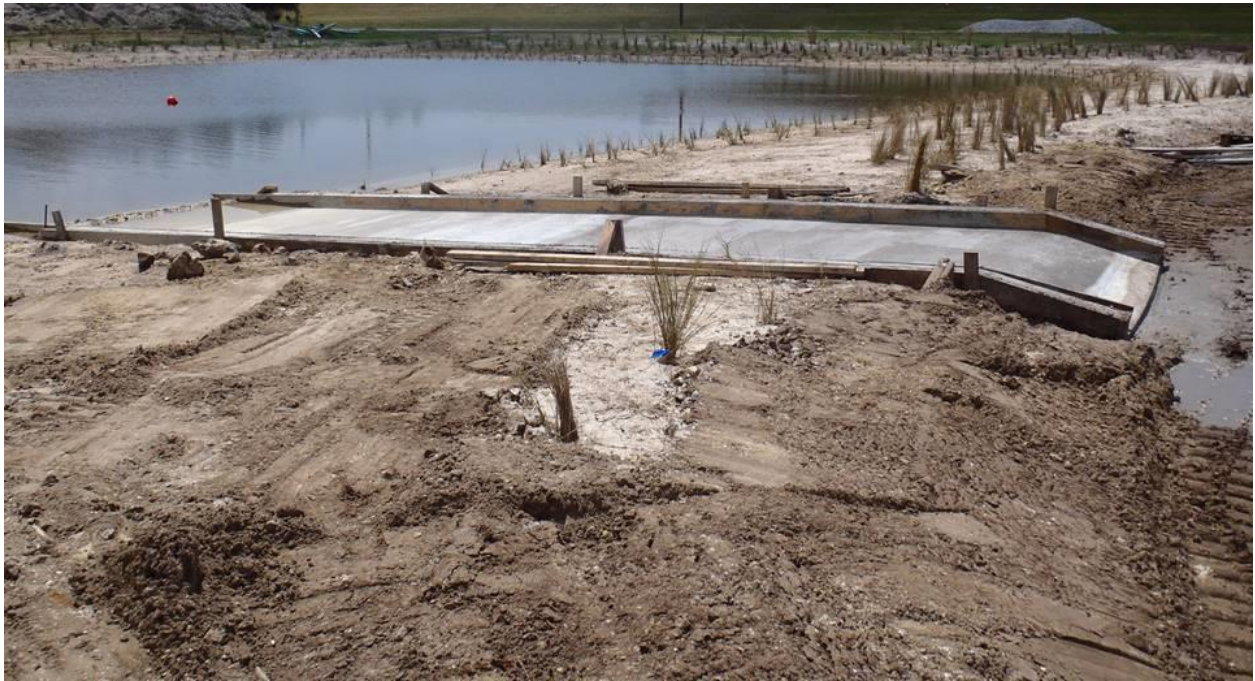
Figure 12 – Concrete Spillway being installed between the marsh and the pond
