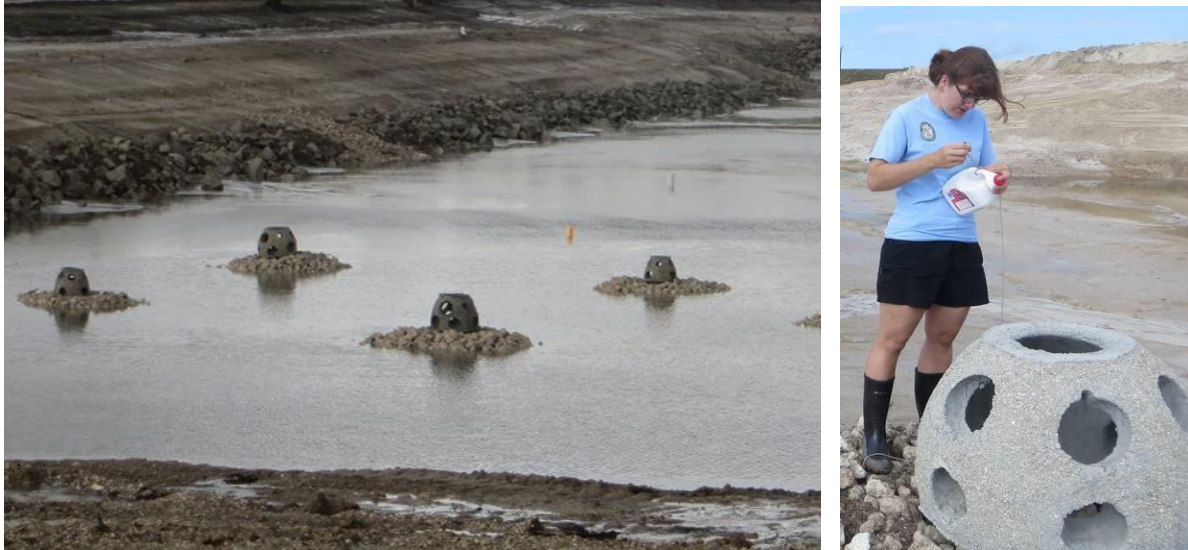
Figure 16 – Some of the concrete Reef Balls located on the pond bottom during construction
