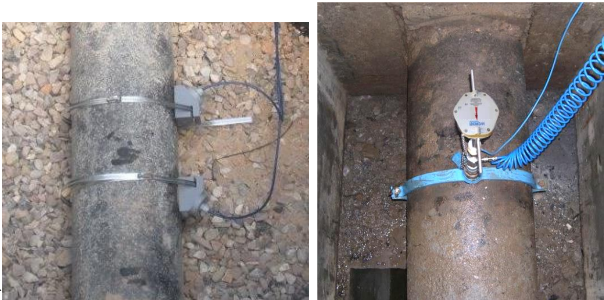
Figure 17: Examples of a strap-on ultrasonic flow meter (left) and a magnetic insertion meter (right), both installed on existing water mains.
