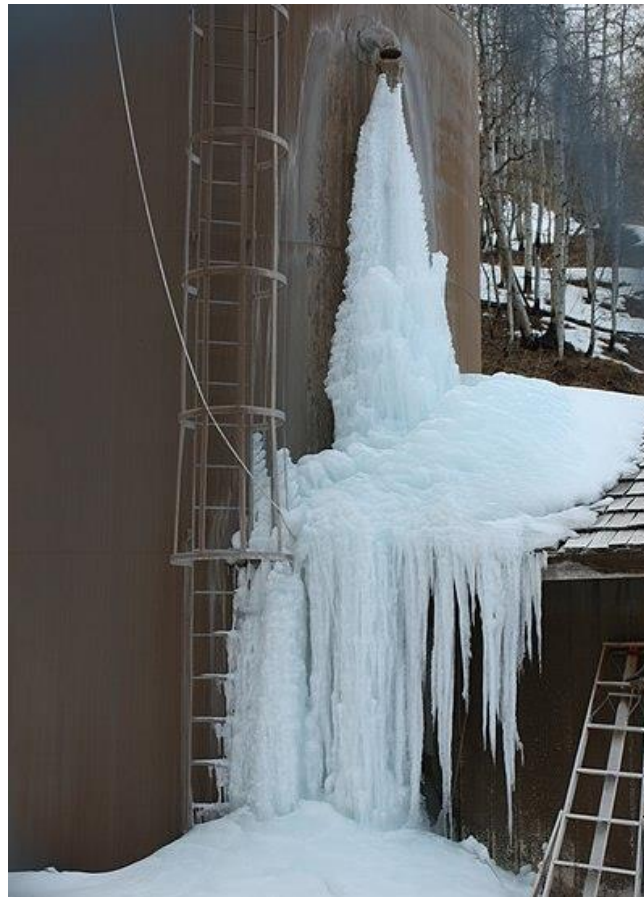
Figure 12: A ground storage tank with an overflow pipe and ice buildup leaving evidence of a recent overflow event.
