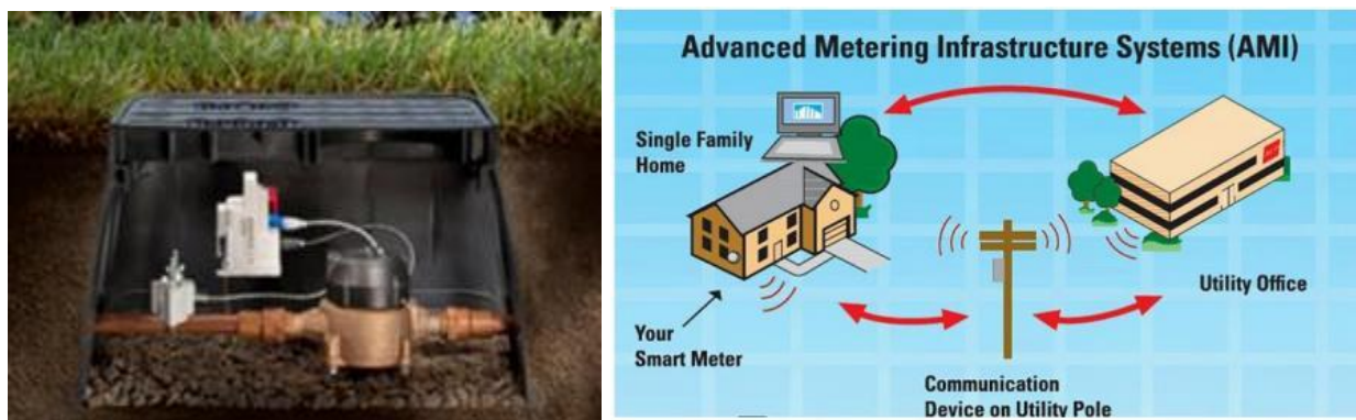
Figure 9: Left: Water meter with AMI communications device in white. Often these radio communications devices will look like hockey pucks on the lid of the meter box. Right: Basic components of an AMI communications system.
