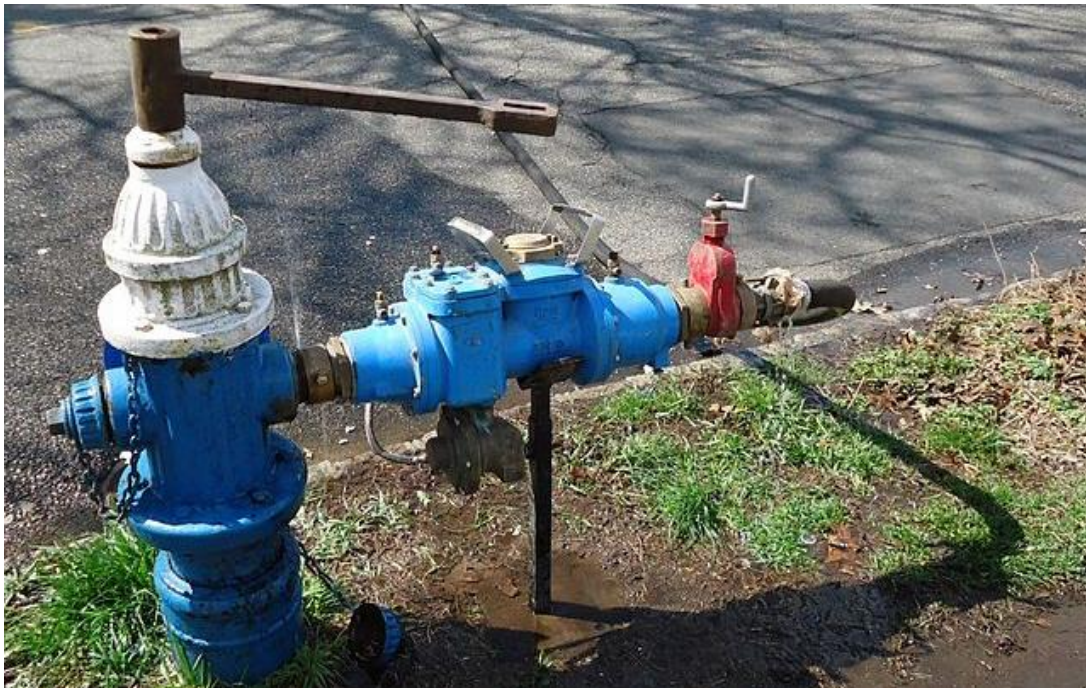
Figure 10: An authorized fire hydrant connection with a flow meter and backflow prevention device. This is an example of unbilled, metered, authorized consumption.
