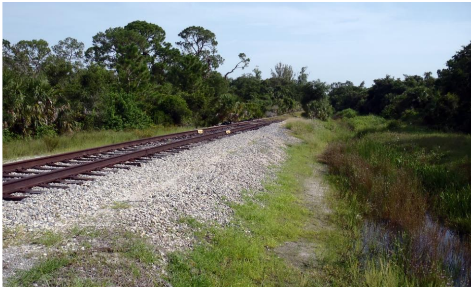
Figure 12 – Railroad drainage ditch to manage stormwater
