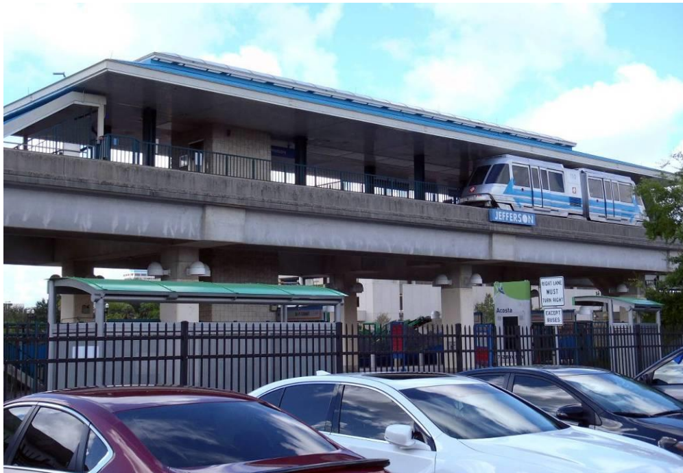
Figure 5 - Elevated Transit Rail Station
