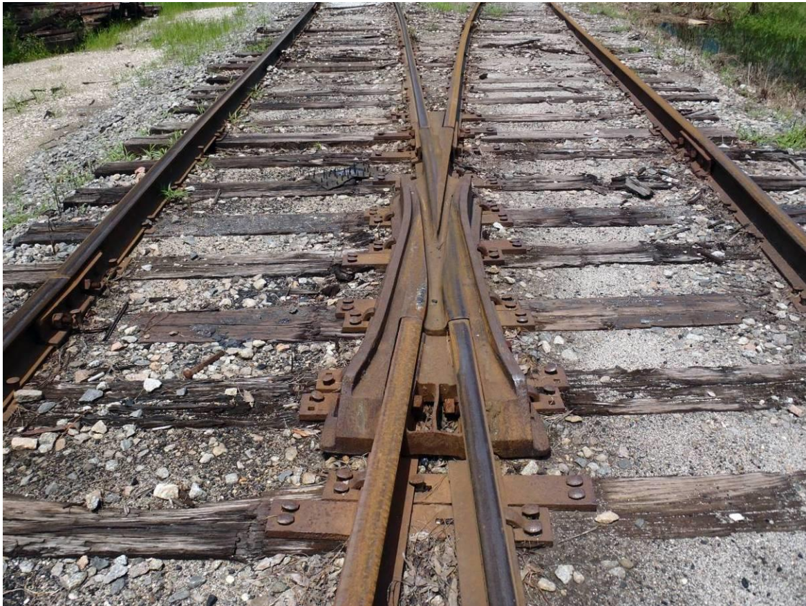
Figure 24 – A frog located at a turnout
