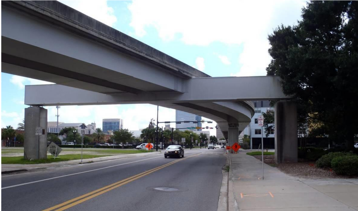
Figure 33 – An elevated commuter rail overpass to avoid an at-grade crossing
