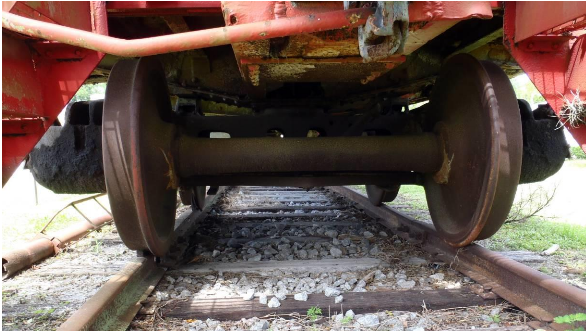
Figure 1 - A rail car's wheels using the standard gauge of 4ft 8.5 inches
