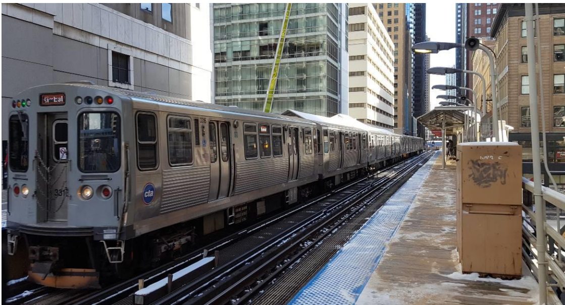
Figure 7 – Elevated transit rail station
