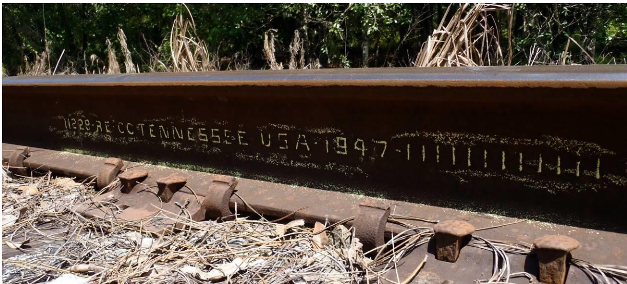
Figure 20 – A 112 pound RE rail manufactured in Tennessee in December 1947 with the stamp highlighted using chalk.
