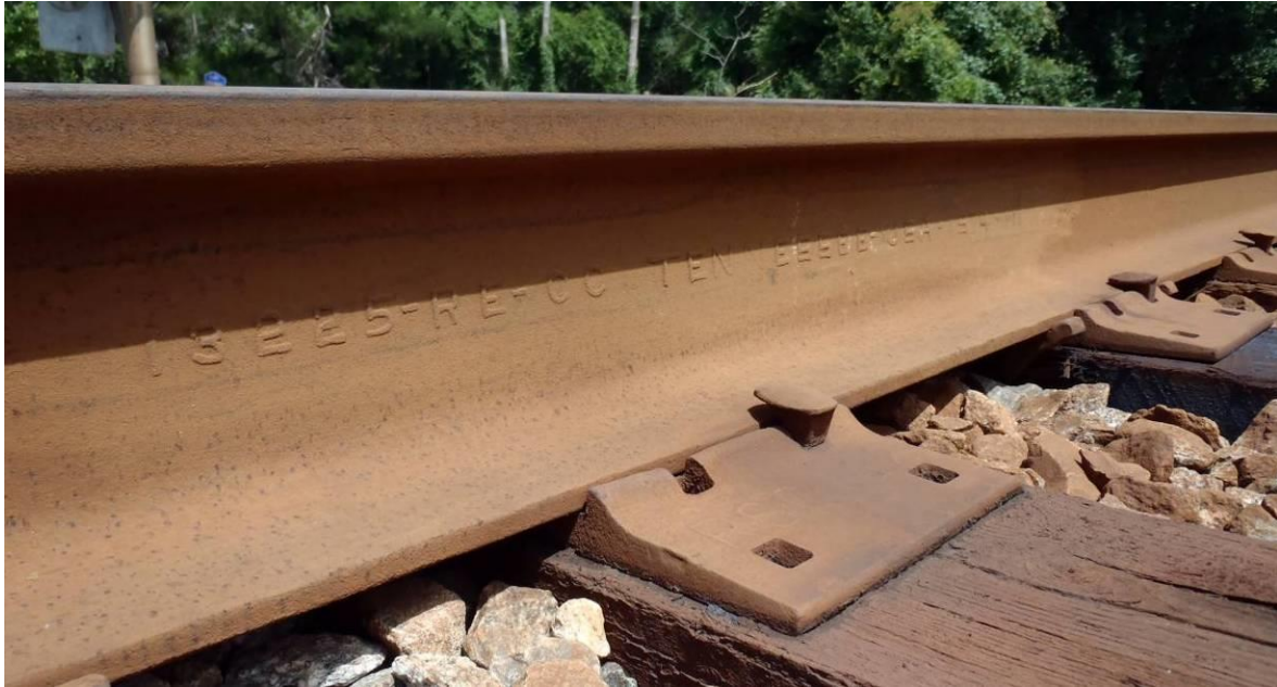
Figure 19 – Rail stamp in its original condition. This one was relatively easy to find because of its good condition. Normally, the stamps are difficult to find because of being covered with rust. This 132 pound RE rail was manufactured in 1974.
