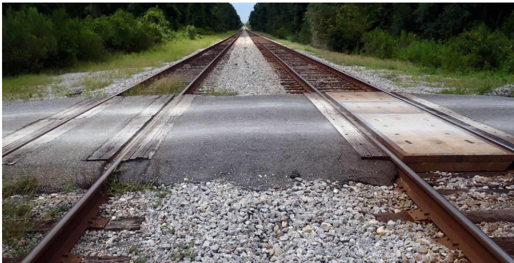
Figure 27 – A rail crossing using asphalt, concrete, & timber materials
