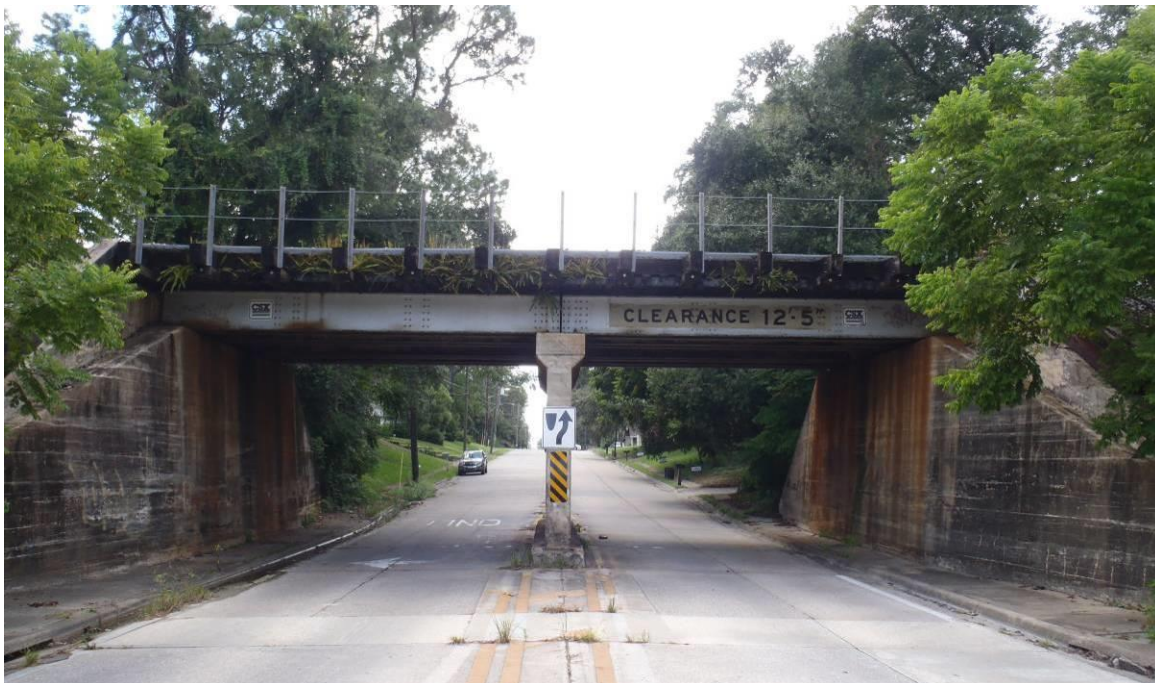
Figure 34 – An elevated road overpass to avoid an at-grade railroad crossing
