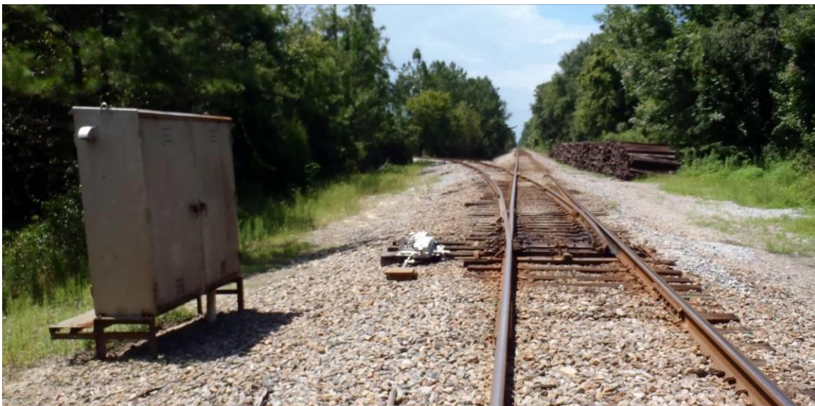
Figure 23 – An electric switch on a rail line
