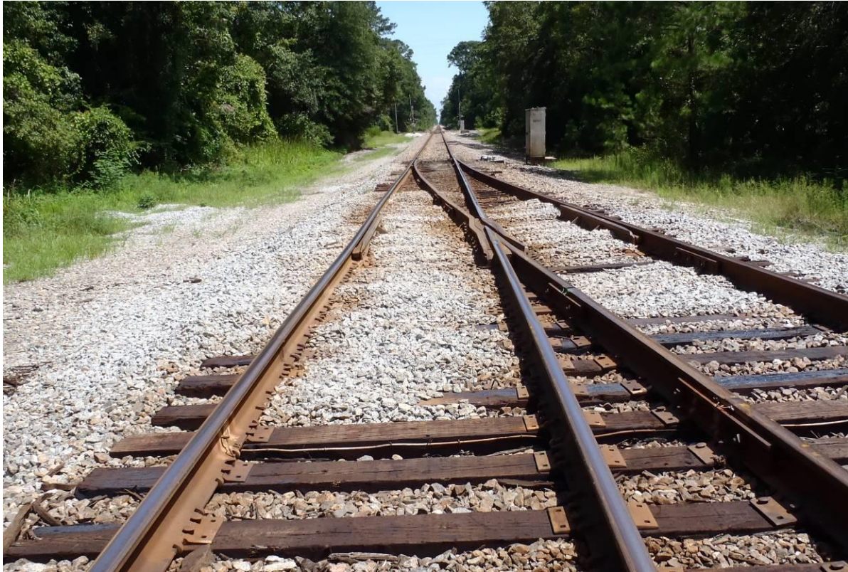
Figure 25 – Another frog showing the geometry of a turnout
