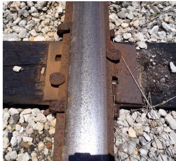
Figure 9 – An installed Tie Plate
