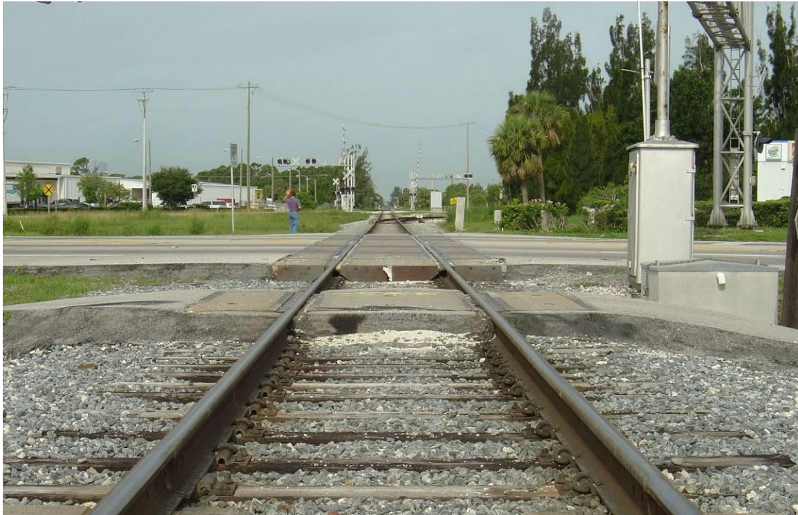
Figure 26 - A road and sidewalk crossing
