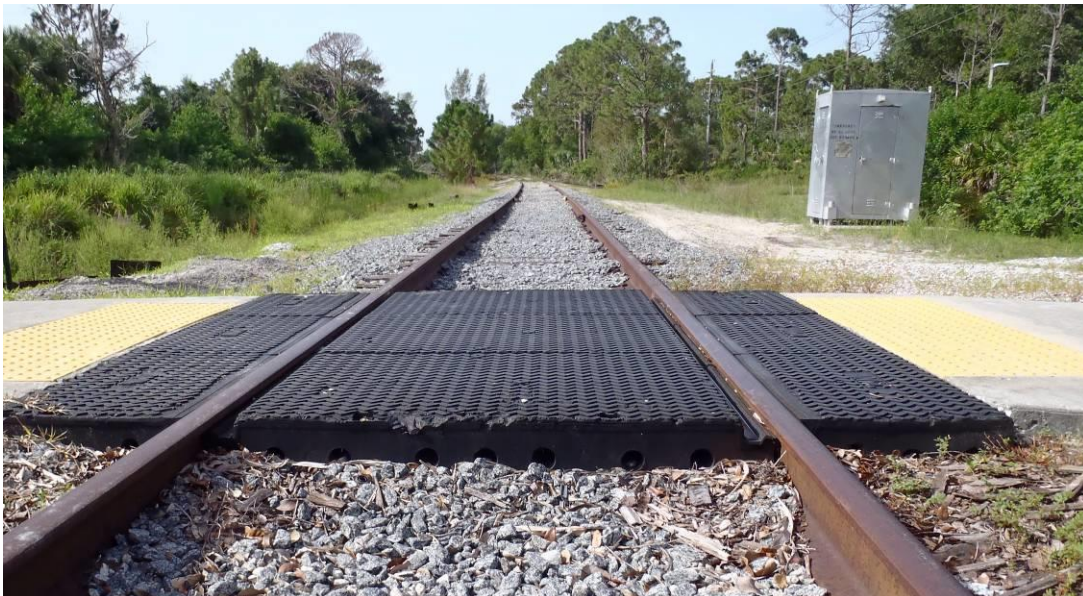
Figure 29 – A pedestrian rail crossing using synthetic materials
