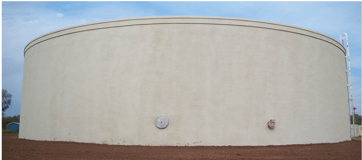
Figure 24: Ground storage tank of concrete construction.
