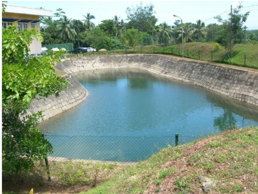
Figure 17: Example of a rainwater storage tank.
