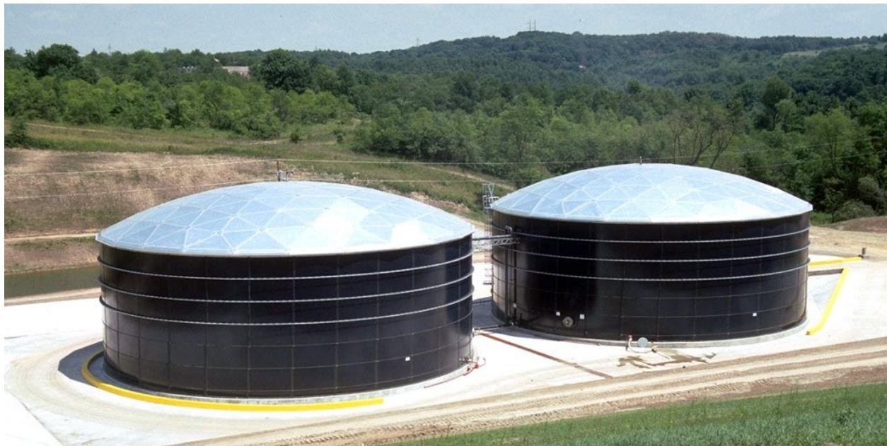
Figure 27: Two ground storage tanks in parallel. Either tank can be taken out of service while the other tank provides the minimum required storage volume.
