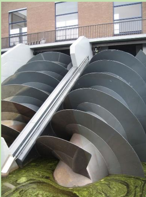
Figure 16: Left: Two single spindle screw pumps with open tops for lifting surface water. Right: Enclosed screw pump with twin screws for high-pressure pumping.
