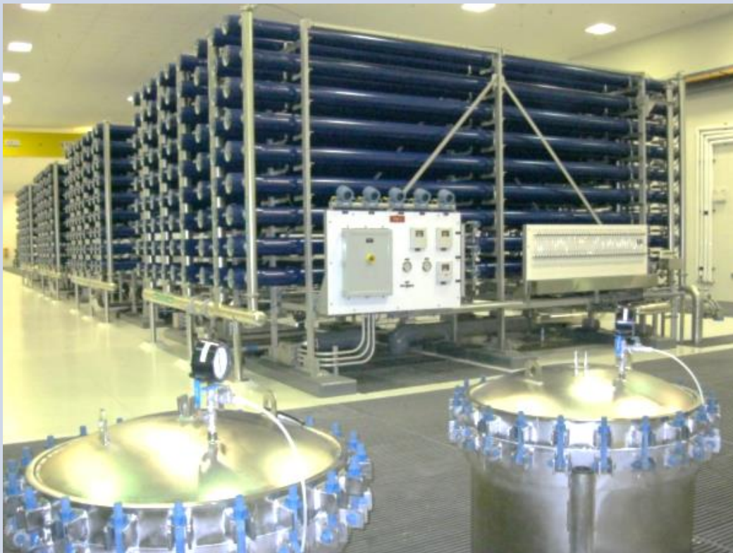
Figure 13: Large water plant with four RO skids, each with (81) blue RO tubes. Two upstream cartridge filters are seen in the bottom.
