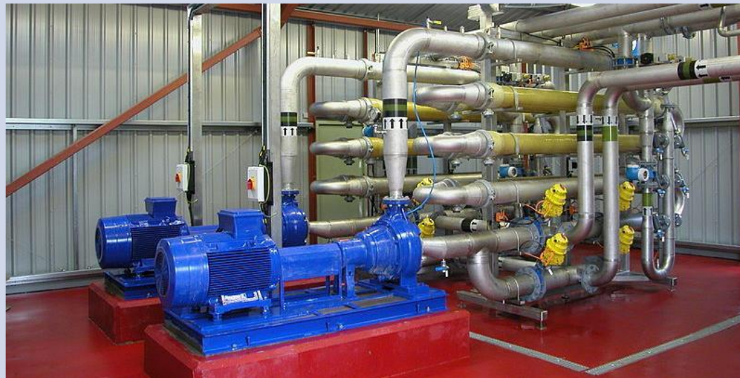
Figure 17: Ultrafiltration membranes (horizontal green tubes) for wastewater treatment.
