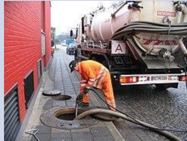
Figure 12: On left, a grease interceptor with major components labeled. On right, a vacuum truck removing the contents of a grease interceptor which serves the red building.
