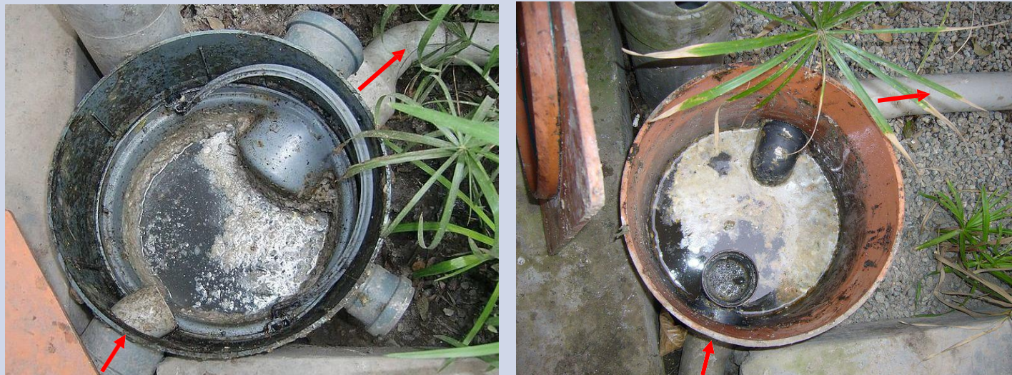
Figure 11: Examples of simple grease traps with flow direction arrows in red.
