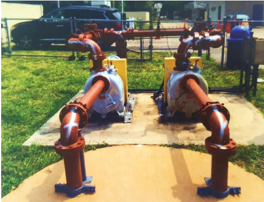
Figure 15: A suction lift station with self-priming pumps mounted on an outdoor slab.
