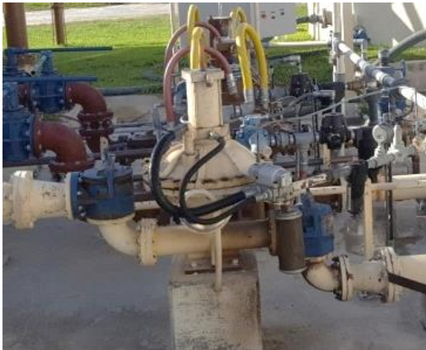
Figure 16: Air diaphragm pumps with compressed air hoses in black, red, and yellow.
