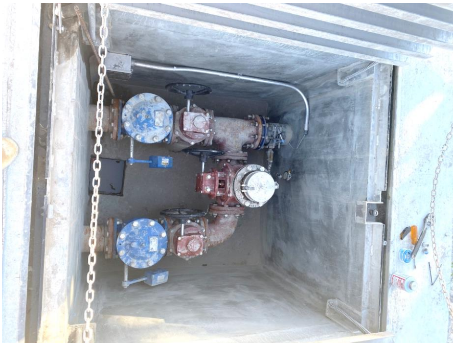
Figure 7: A valve vault with two check valves (blue), plug valves (red), a pump-out connection on a riser, and a pressure gauge on the force main (to right).
