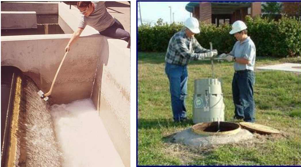
Figure 14: Poorly chosen sample location due to safety concerns (left), and inspectors setting up a composite sampler at a discharge/sample manhole (right).
