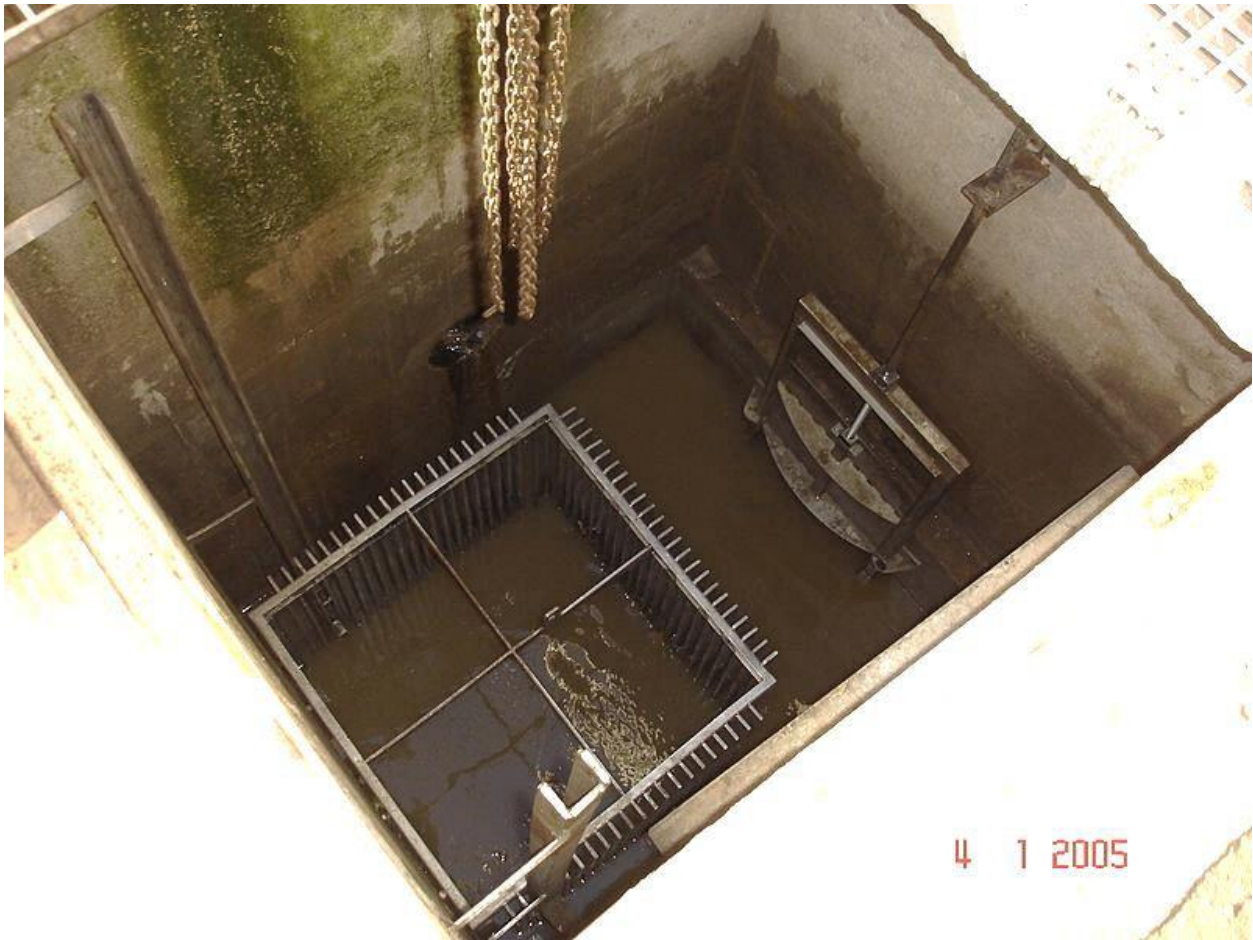
Figure 2: Example of a wet well with a basket screen, as part of a small industrial pretreatment system with primary treatment.
