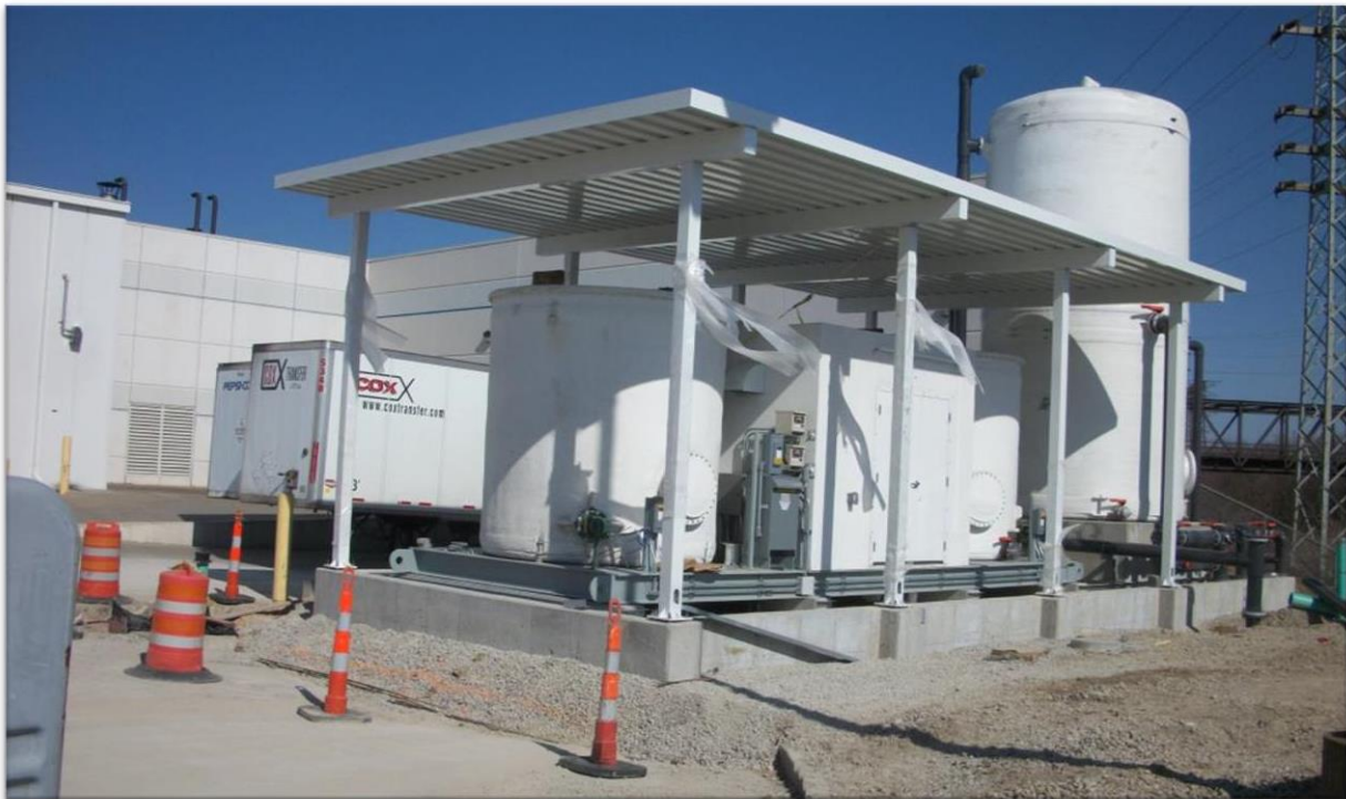
Figure 5: Example of a manufacturing facility with a pretreatment system circled in white (top) and at ground level (bottom). The system includes a large equalization tank and a pH neutralization system.
