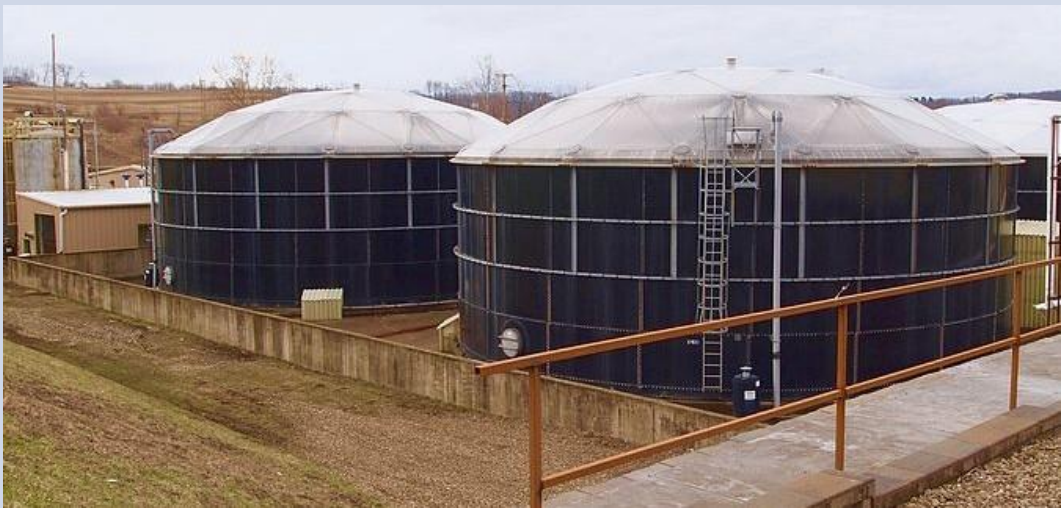
Figure 8: Two 400,000 gallon equalization tanks for landfill leachate pretreatment. Source: commons.wikimedia.org/wiki/File:Leachate_processing_tanks.jpg, Z22, CC-BY-SA-4.0
