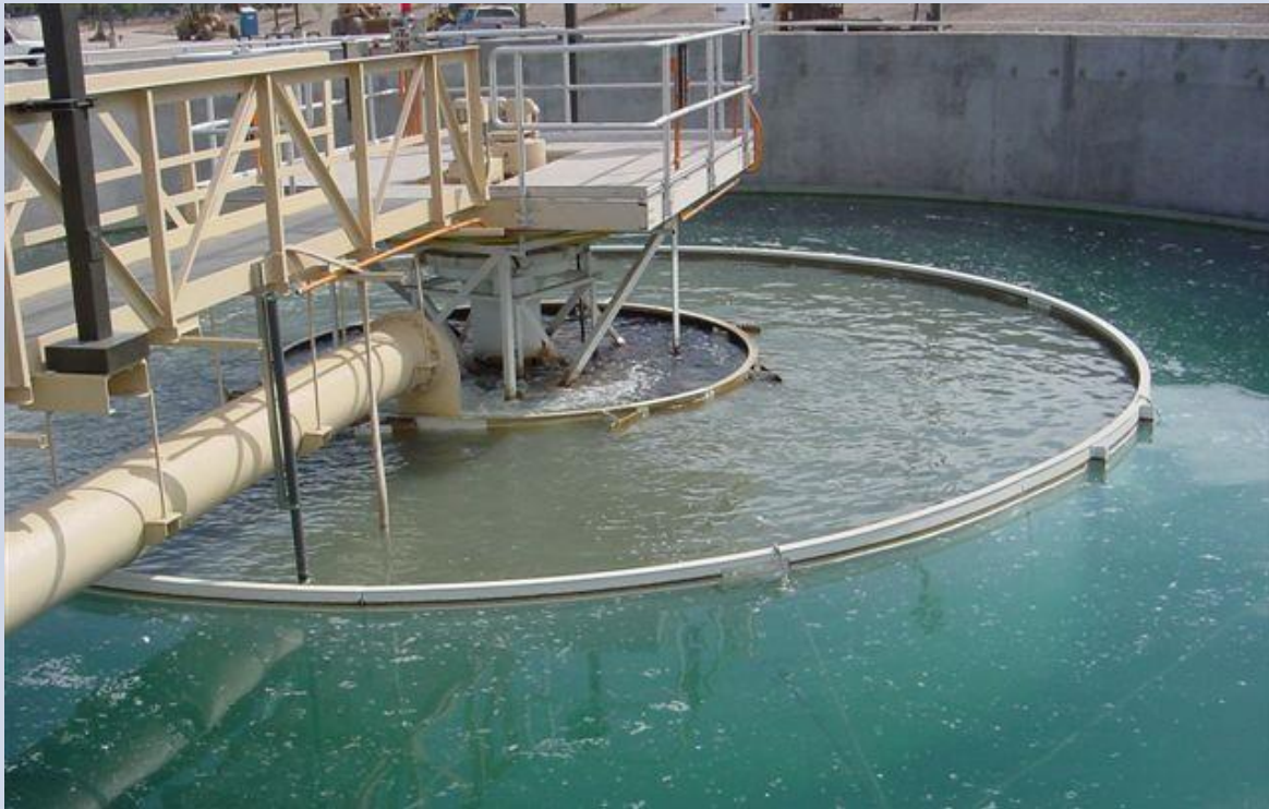
Figure 21: Example of a flocculation well/zone in a circular clarifier. Polymer can be added to the influent pipe to encourage flocculation in the well.
