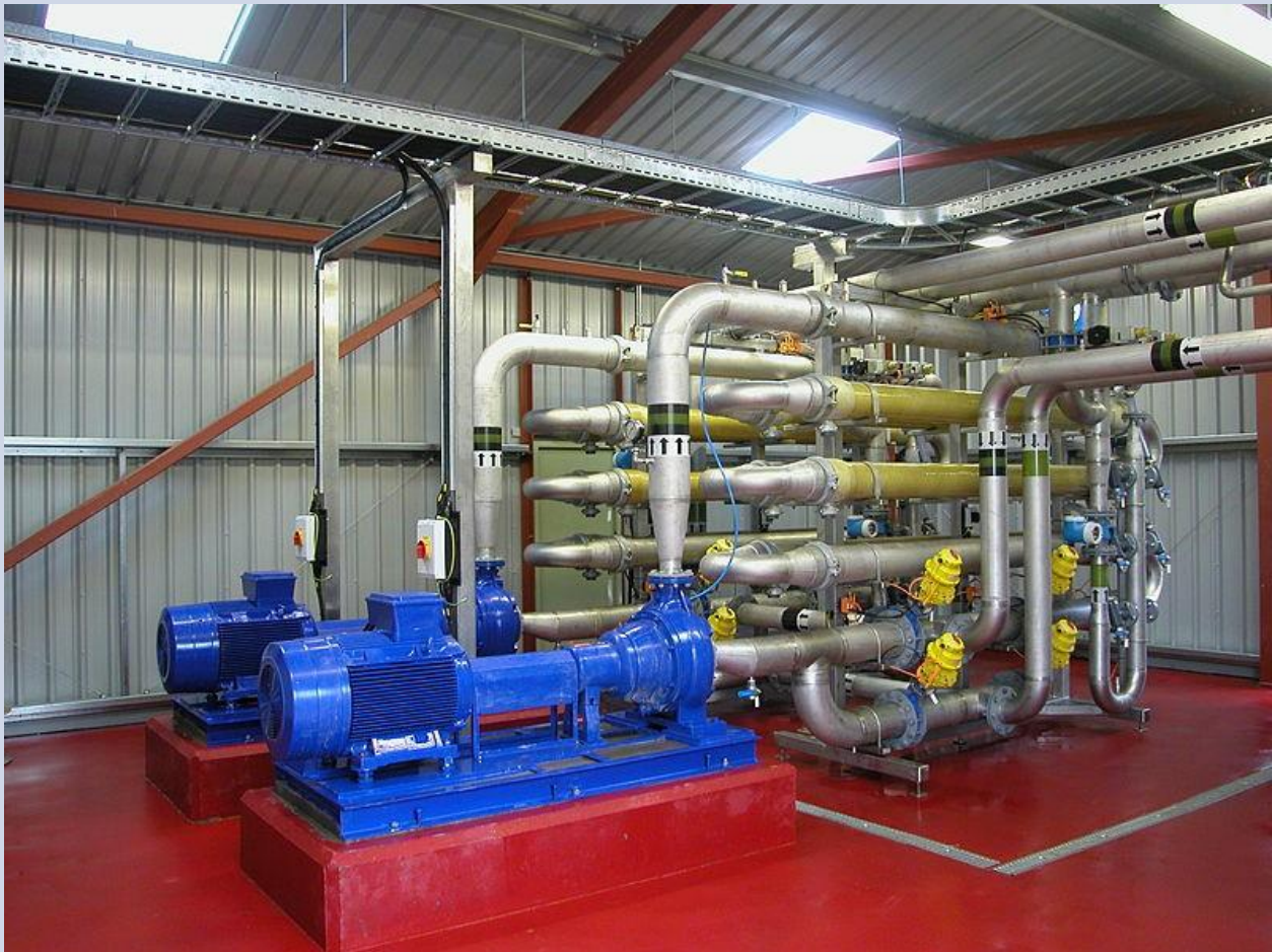
Figure 13: Ultrafiltration membranes (horizontal green tubes) for wastewater treatment.
