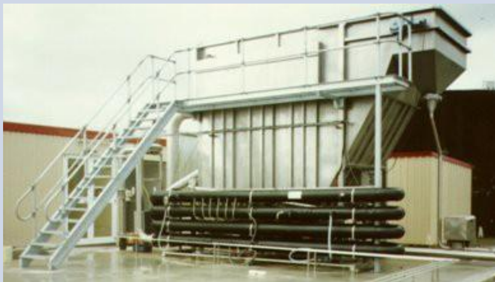
Figure 11: Example of a DAF system. Air is added to the influent and small air bubbles form and attach to oil and suspended solids, floating them to the surface where they are skimmed off as solids. DAFs are common at oil refineries, chemical plants, and paper mills.
