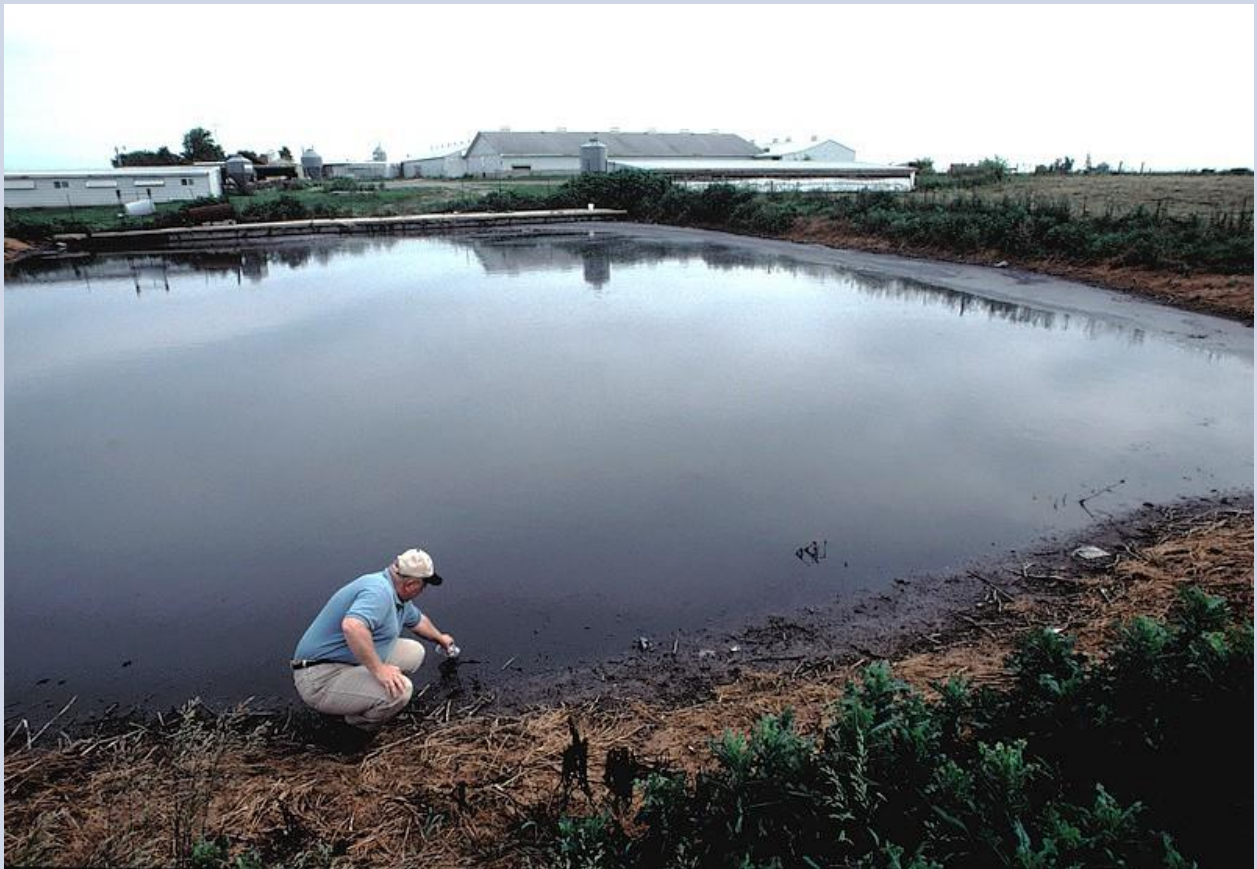
Figure 29: Operator taking a sample from a wastewater lagoon at a hog farm operation. Earthen basins require composite liners to isolate from groundwater. Settled sludge is to be removed periodically.
