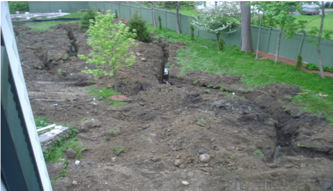
Figure 6 See how trenching avoids the roots of a mature tree.
