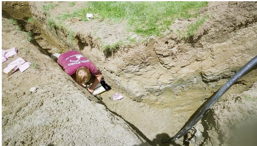
Figure 7 Footing drain space with Loop below and pink foam board insulation. Note that the worker only enters the < 5ft. deep trench after it is partially backfilled.
