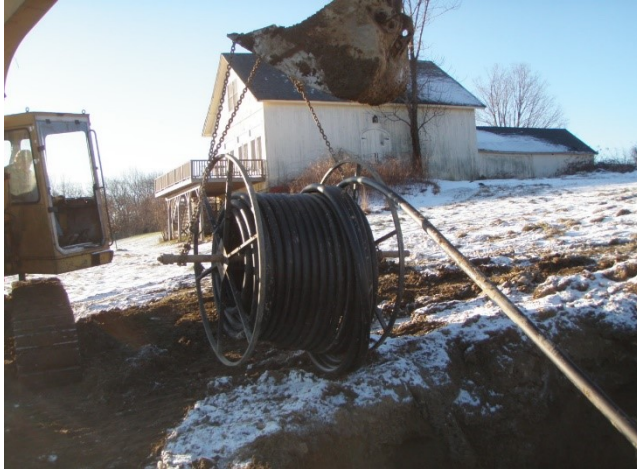
Figure 12 2in. diameter single HDPE loop pipe is unwound from 4ft. wide spools and installed by excavators.
