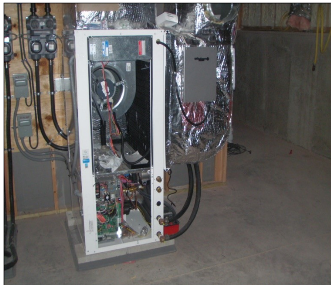
Figure 22 New home unit heat pump with compressor on bottom and air handler on top.
