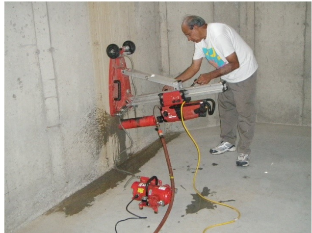
Figure 28 Wet drilling with drill attached to wall by suction.
