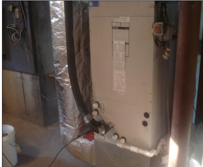
Figure 21 Retrofit split air handler and ductwork with heat pump refrigerant in black insulated copper line.
