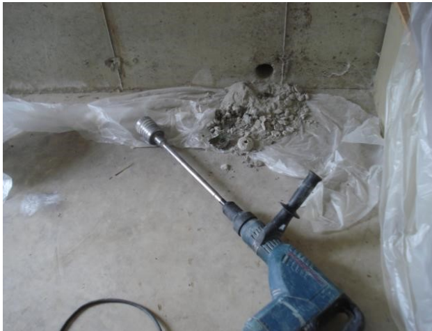
Figure 27 Dry drilling that creates concrete dust.
