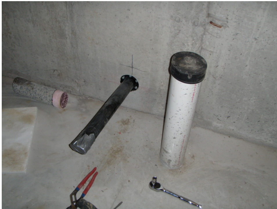
Figure 29 To drill through an existing concrete or block foundation wall, select a drill bit that is correctly sized for the outside loop diameter and the Link Seals that will be used to waterproof everything. Pictured here, six Link Seal bolts for 2in. HDPE loop tightened by ratchet and core with pink insulation to the left.
