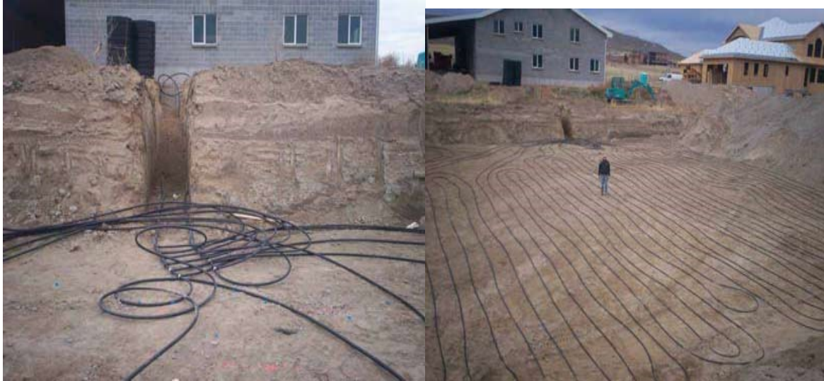
Figure 16 Complete dirt removal versus trenching. ( http://www.geoexchange.org/ )
