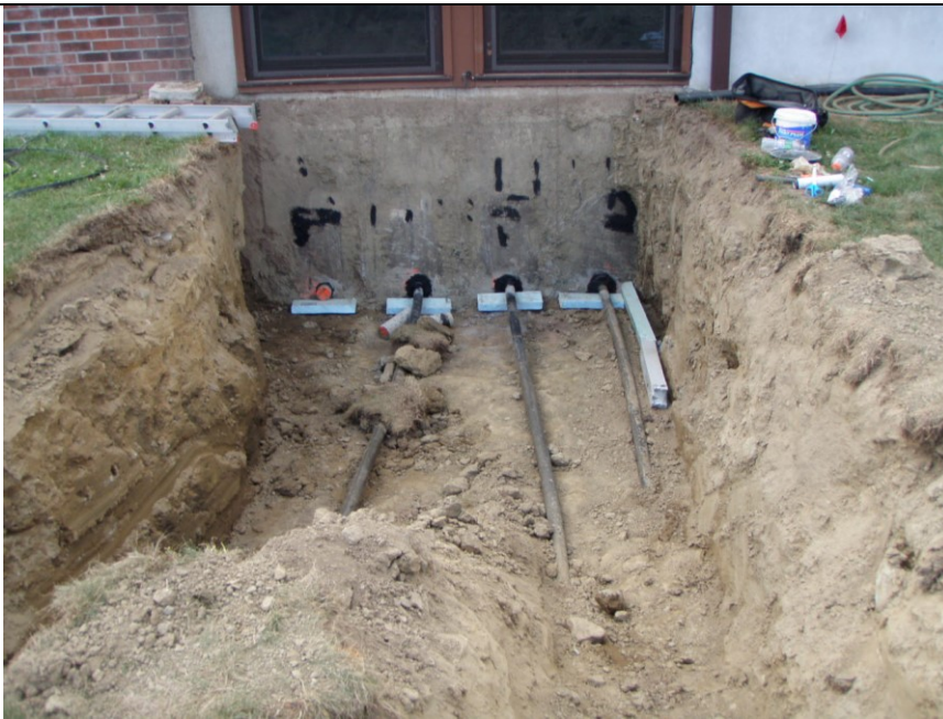
Figure 30 Inlet and outlet loop insertions into basement.
