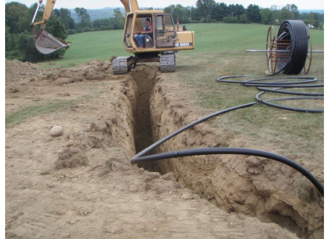
Figure 12 2in. diameter single HDPE loop pipe is unwound from 4ft. wide spools and installed by excavators.
