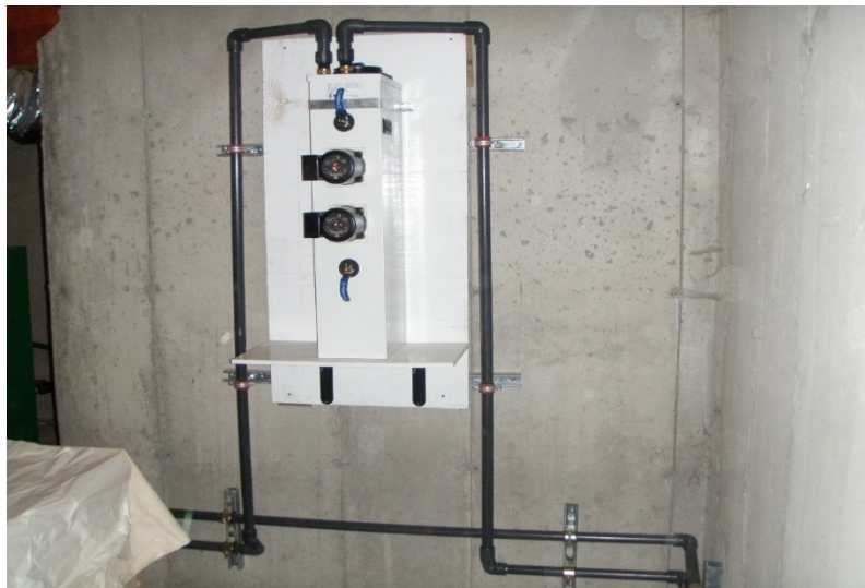
Figure 20 In this alternative flow control center, a non-pressurized canister circulates loop water and PG to the heat pump at about 3-5 psi.
