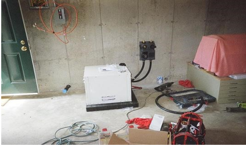
Figure 19 Under assembly: 2 in. loop inlet with blue cap, 2.5-ton split heat pump. The flow controller Grundfos pump is wall mounted. HVAC contractor will complete connections once the loop outlet is pushed through the second drill hole. Electric power whip, upper left.
