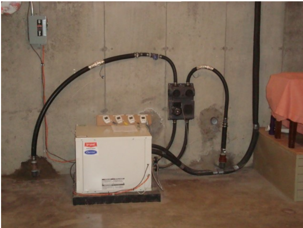
Figure 31 Working split unit heat pump with flow center accessing loop inlet and outlet. A short reserve loop installed 24in. above the slab was not necessary. The line to the ceiling is insulated copper carrying refrigerant to the air handler.
