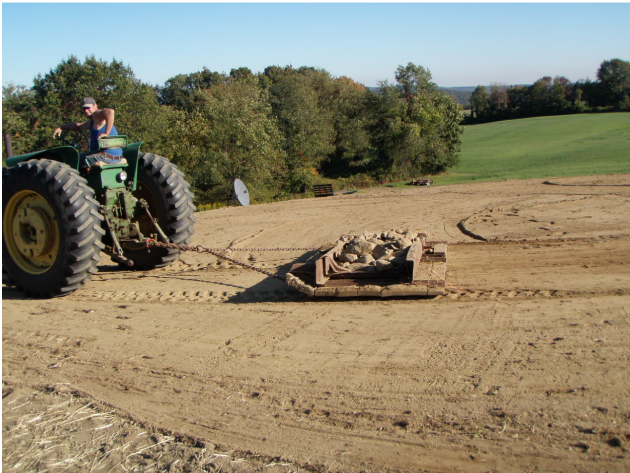
Figure 33 Using weight to compact backfilled mounds in a loop field.
