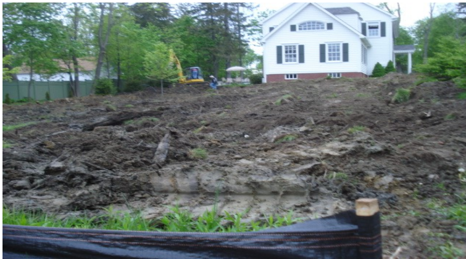
Figure 8 Silt fence erosion control.
