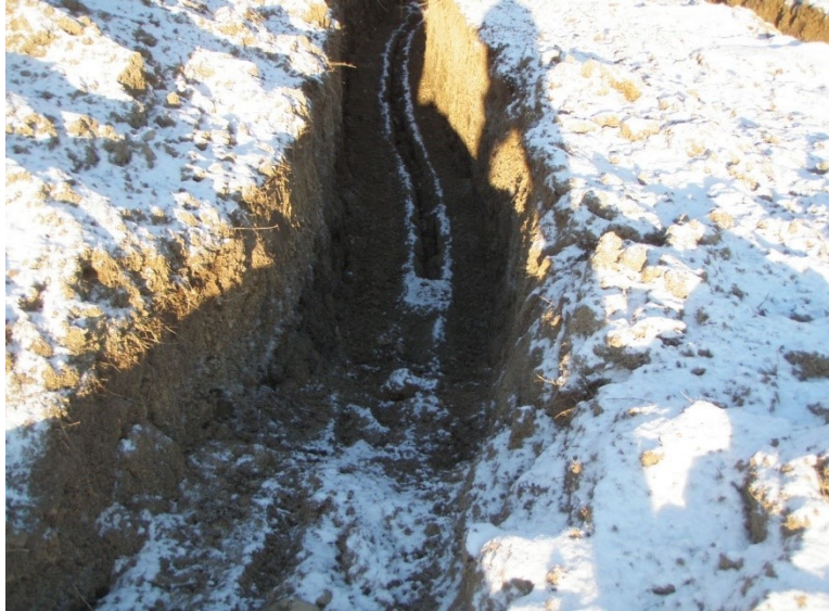
Figure 15 A 4 in. wide Ditch Witch trench at the bottom of a 5 ft. deep excavated OSHA trench.
